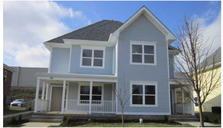
New rental housing in Davis Park included two duplexes with a farm-house design made with clap-board style fiber cement siding with small porch entries on each side of the building. © 2004 Juliana McDonald.
