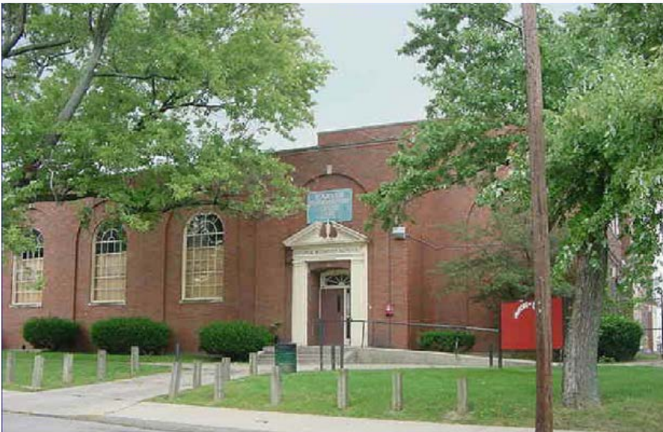
Carver Center on Patterson Street, formerly the George Washington Carver Elementary School.
