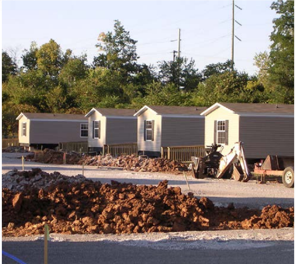
Sixteen manufactured homes were placed in Southend Park as interim housing. Residents moved into interim housing in 2008. Each home came with all appliances, including a washer and dryer. Residents were not required to pay rent or necessary utilities as they prepared for their move into replacement housing.
