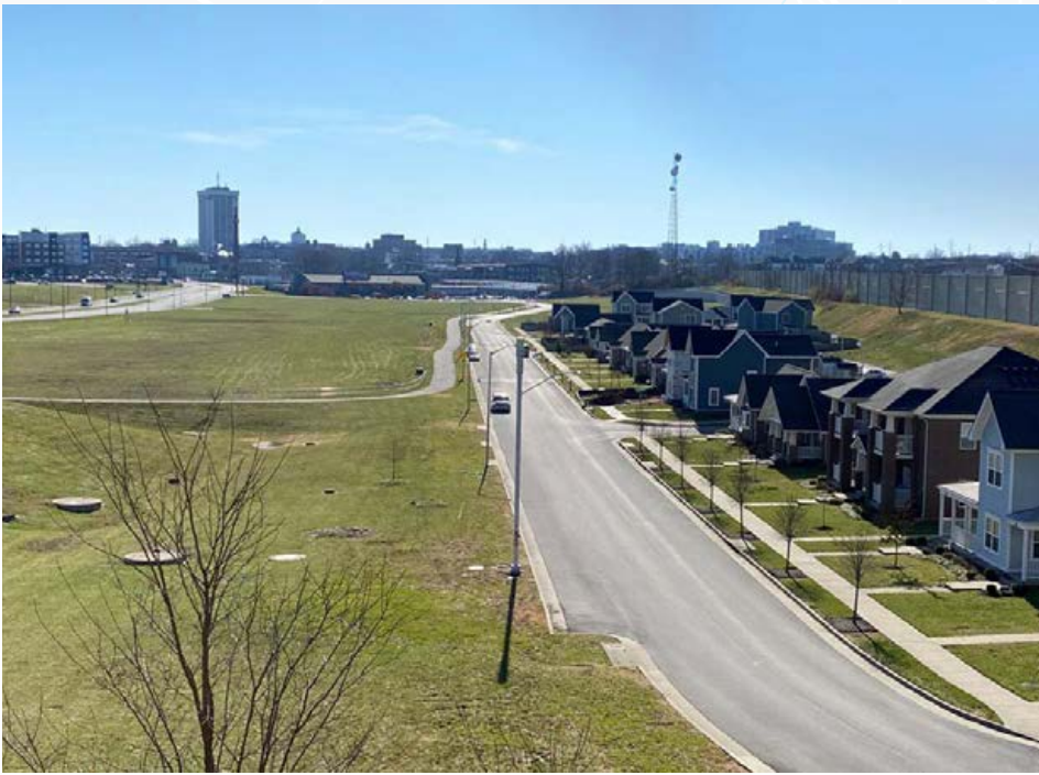
Oliver Lewis Way (part of the NPEP corridor) at the far left photographed from the West High Street viaduct. Oliver Lewis Way connects Newtown Pike to South Broadway. The UK's Patterson Tower can be seen in the background. On the right, rental units and individually owned homes in Davis Park can be seen. This housing was created by the NPEP and the LCLT to replace previous homes in DB (a neighborhood dating back to 1865).
