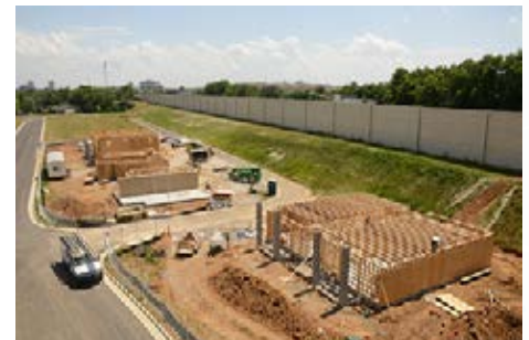
New rental units under construction during Phase I of the NPEP.
