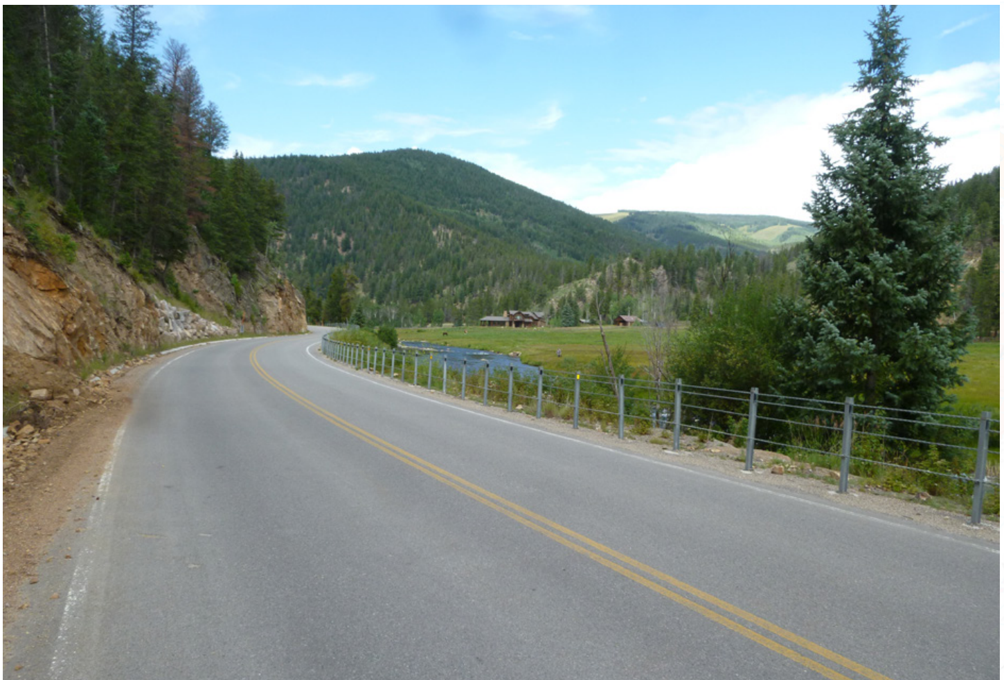
Cable barrier used along a roadside in Gunnison County, Colorado.
