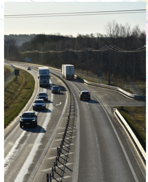
This is an example of a 2+1 road in Sweden.
