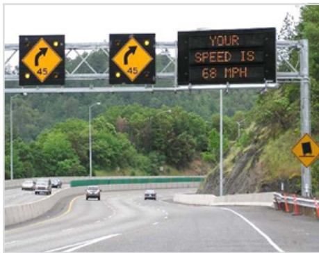
Speed feedback signs like this one can encourage drivers to follow posted speed limits and advisory warnings.
