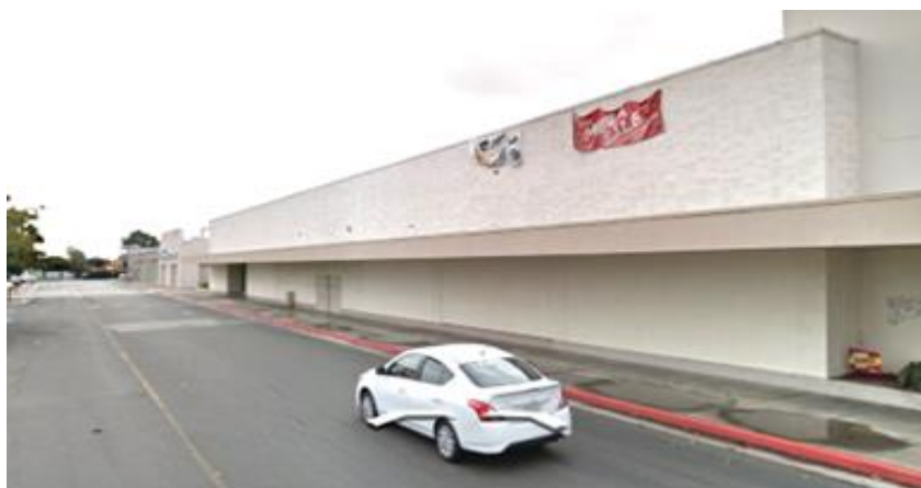
Figure 2. Southland Mall. Photo from Google Earth (7/14/22)
