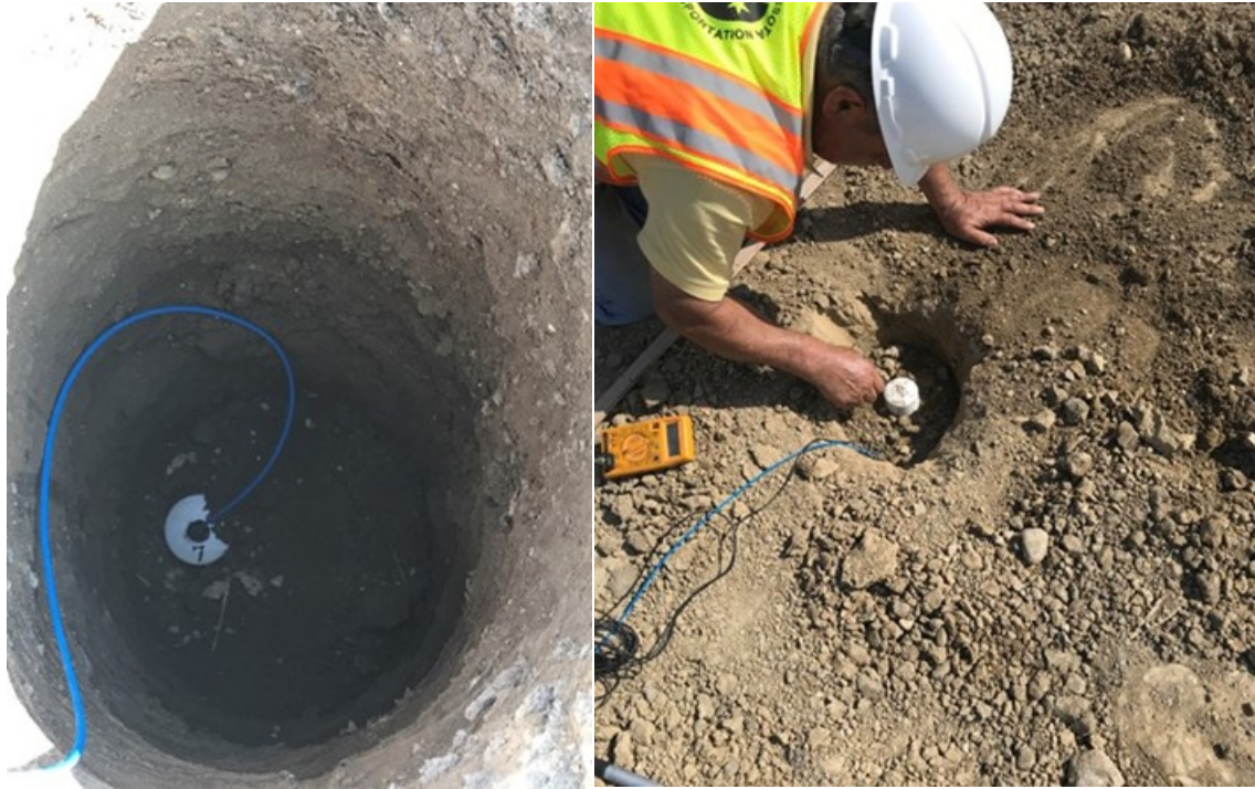
Figure 16. Instrumentation of the geophones in the subgrade.
