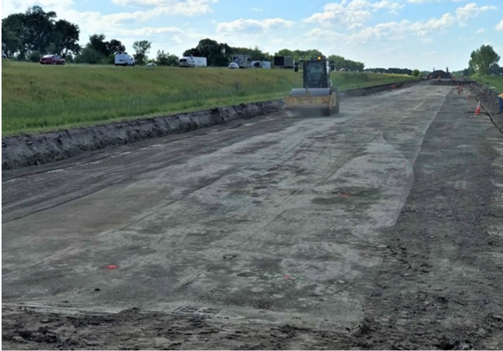
Figure 19. IC Pre-Mapping Subgrade.
