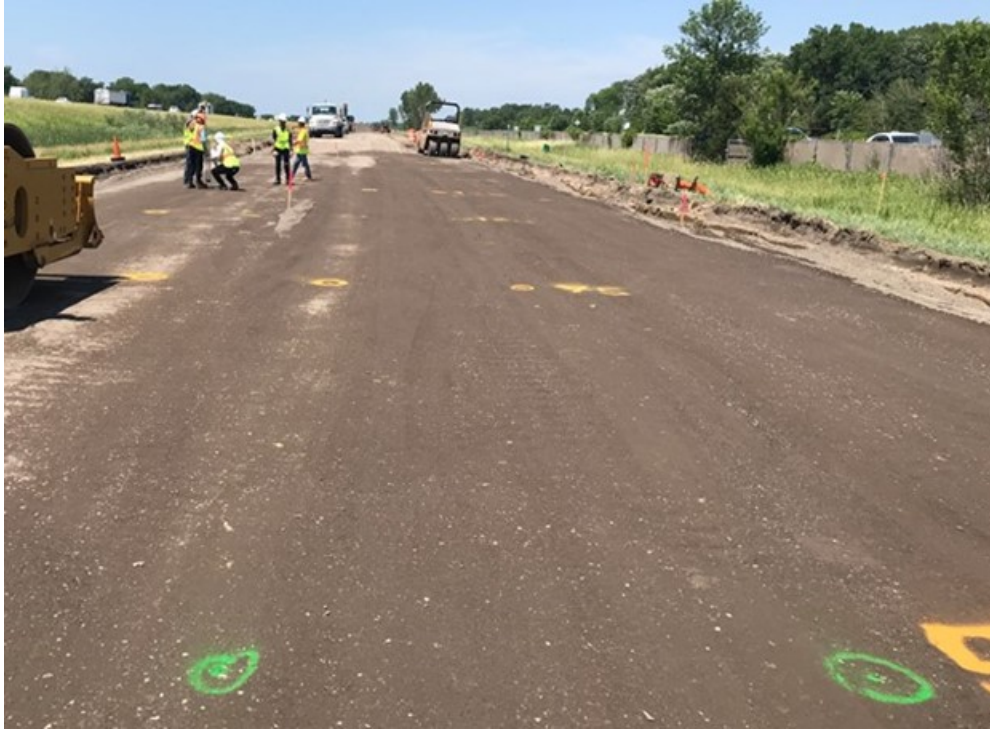
Figure 21. Test Cell Markings for Spot Tests on Subbase.
