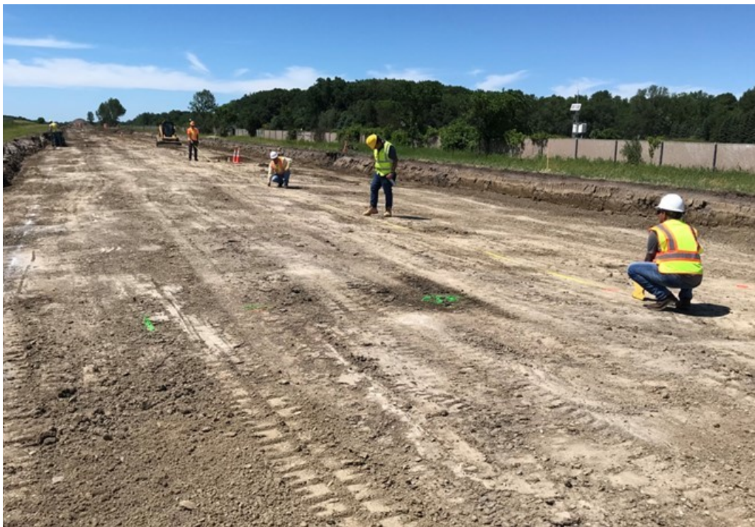
Figure 12. Test Cell Markings on Subgrade.
