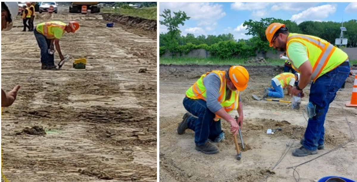
Figure 25. NDG Density and Moisture tests and Soils Sampling.
