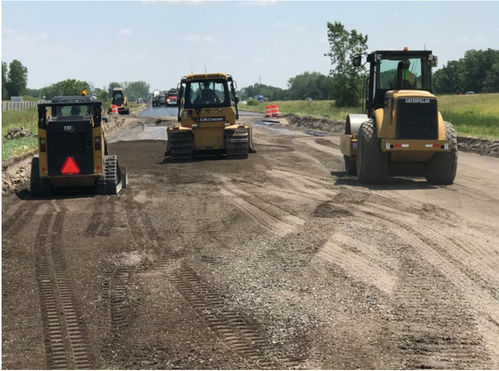
Figure 20. Placing and Compacting the Subbase Layer Materials.
