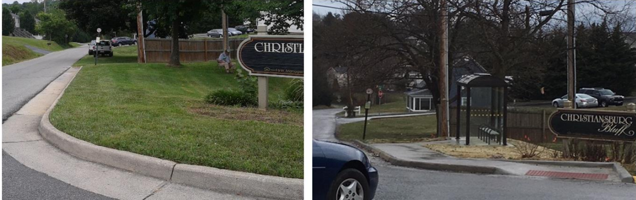
Figure 3. BT Stop 2101: Before (left) and After (right) Installation of Solar Shelter With Bench, Concrete Pad, Sidewalk, and Intersection Curb Ramp. Images by Erik Olsen of BT.
