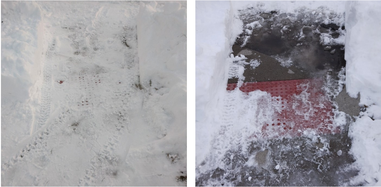
Figure 2.4 Curb ramp immediately after snow removal (left) and one day later with refreeze beginning to occur at bottom of ramp. (Source: John Shaw/Iowa State University)
