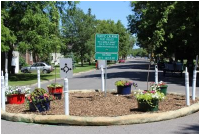
Figure 3.1 Bio-Log roundabout. (Source: Jacob Reuter/MnDOT)
