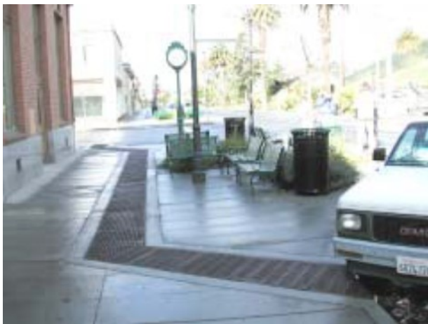
Figure 5.2 Drainage channel through a curb extension, bridged by drain grates. (Source: San Diego Association of Governments)
