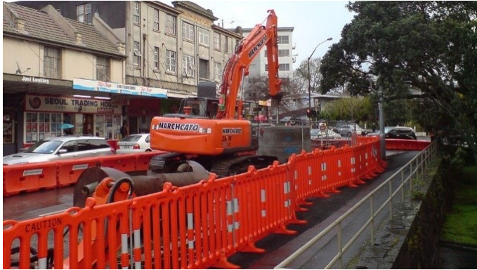
Figure 5.4 Pedestrian walkway delineated by prefabricated fence panels. (Source: Ingolfson/Wikimedia Commons)
