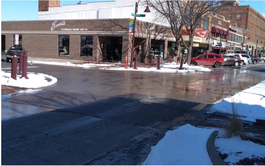
Figure 2.7 Tight corner radius combined with use of bollards and stamped concrete crosswalk. (Source: David Veneziano/Iowa State University)
