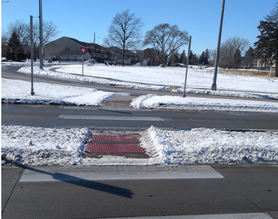
Figure 5.3 Cut-through design for pedestrian walkway across a roundabout splitter island in Ames, IA. (Source: David Veneziano/Iowa State University)
