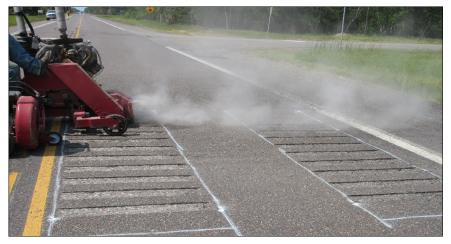
Rumble strips milled into pavement can be filled in later, if necessary. Also, placing the strips closer to the centerline than to the road's edge can encourage drivers who choose to maneuver around the strips to move away from the opposite lane toward the road's shoulder.
