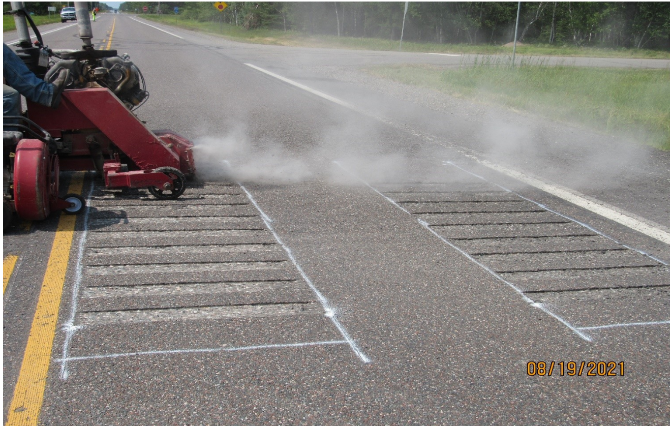
Figure 2-2. Transverse rumble strips being milled in
