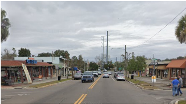
Figure 2. Photo. A roadway segment on SR 21 before improvement.
