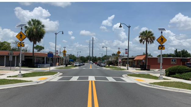
Figure 3. Photo. A roadway segment on SR 21 after improvement.
