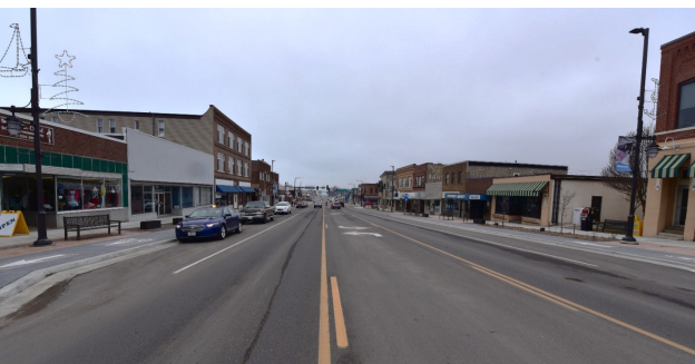
Figure 3. Photo. A roadway segment on MN 28 after improvement.
