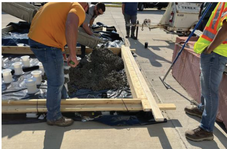
Figure 5.9 Concrete casting of the slab of Shelby field testing.
