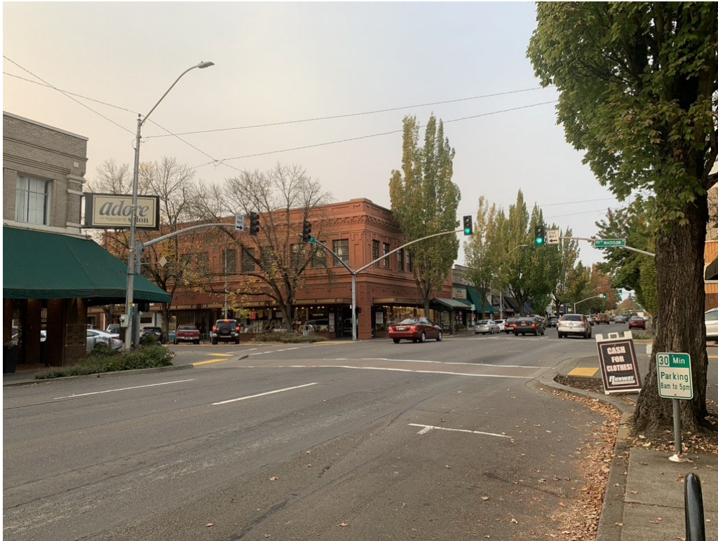
Figure 2.3: Curb extension example at intersection
