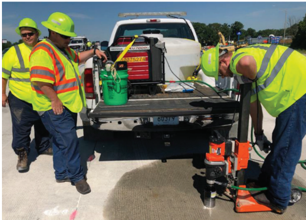
Figure 3.8 INDOT typical core drill equipment.
