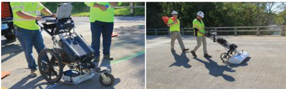
Figure 2.2 Example of ground-coupled GPR equipment.
