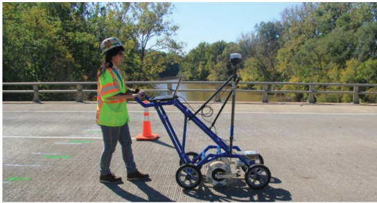
Figure 2.4 Example of IE equipment.
