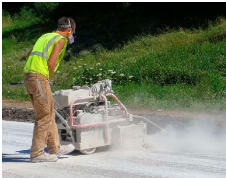
Performing an early-entry saw cut
