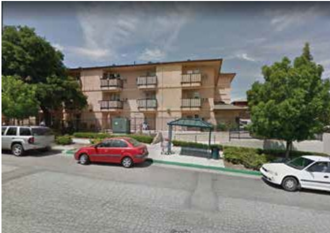
Fence around Chet Dotter at front allows for bus stop access.
