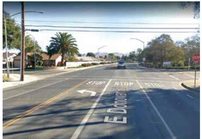
Intersection of Suey Road and E. Donovan is a four-way stop with parallel bar crosswalk instead of high visibility crosswalk.
