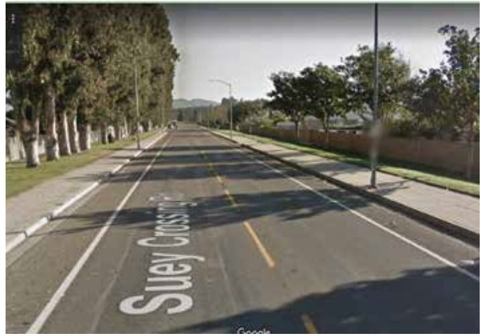
Wider sidewalks and a bike lane help buffer pedestrians from motor vehicle traffic on Suey Crossing Road.
