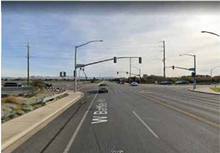
Minimum width sidewalks and bike lane along Battle Road lead to large intersection. LRSP identifies crashes at this intersection and mid-block.
