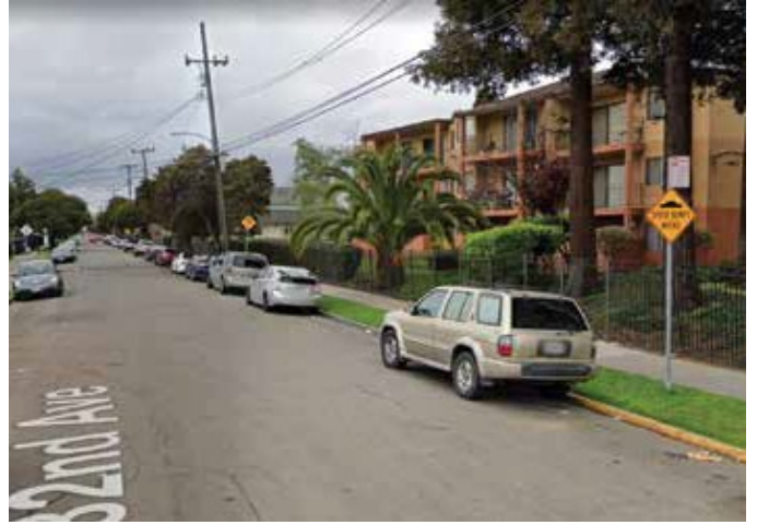
Sidewalks along 82nd Avenue are generally in good repair. Speed bumps and a posted speed 15 MPH speed limit are intended to create comfortable walking conditions.
