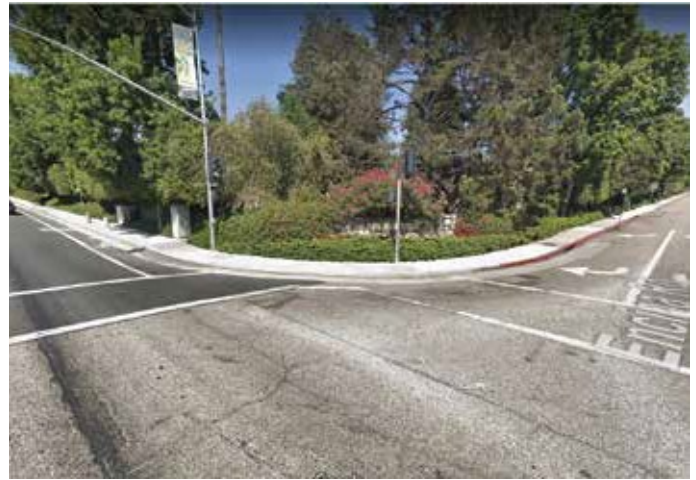
Wall and fence around portion of perimeter constrains bus stop access.
