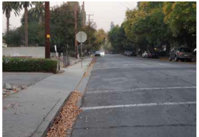
Intersection on Harrison leading to Larking Park Community Center lacks curb ramps and some crosswalks. However, the crosswalk does not align with driveway, intended as a curb ramp.
