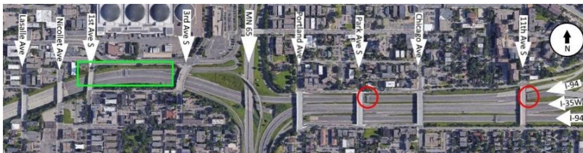
Figure 2-1 Aerial view of implementation site.
