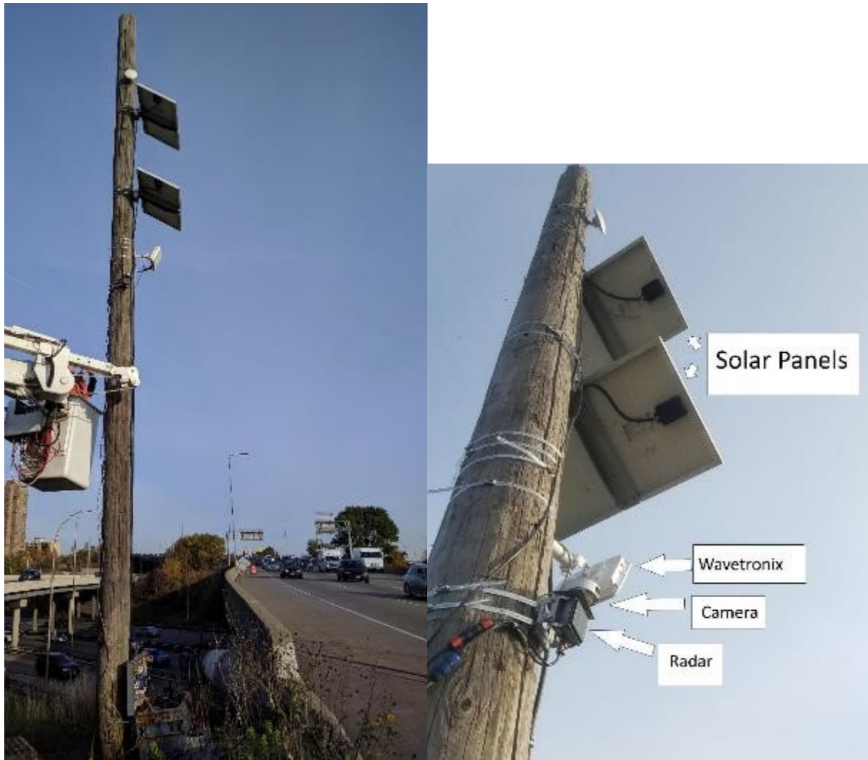
Figure 3-5 Hiawatha station being assembled.
