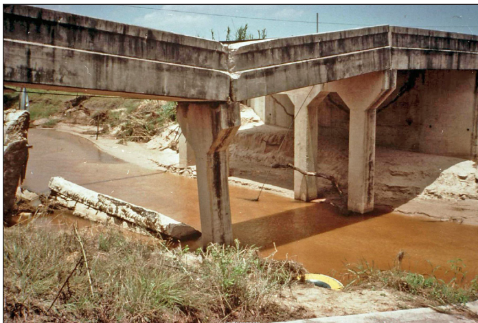
Bridge failure due to scour.
