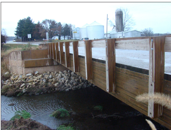
Figure 1. Glulam girder timber bridge in Buchanan County, Iowa. (Photo credit: Zach Carnahan)
