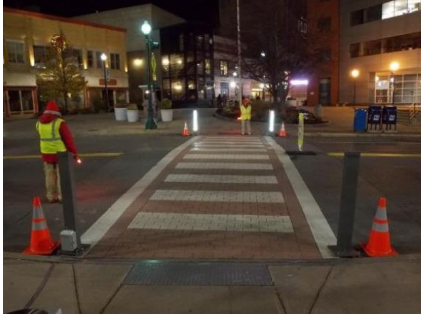
Figure 3. Image. Bollard crosswalk lighting system at night [8]
