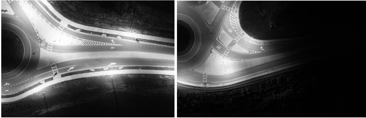
Figure 58. Photo. Roundabout approaches with uniformity levels <3:1 and >3:1 respectively.
