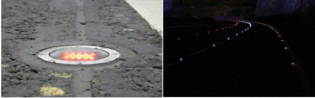
Figure 8. Image. Actively illuminated road studs with nearside red studs, center-line white studs, and offside amber studs [29]
