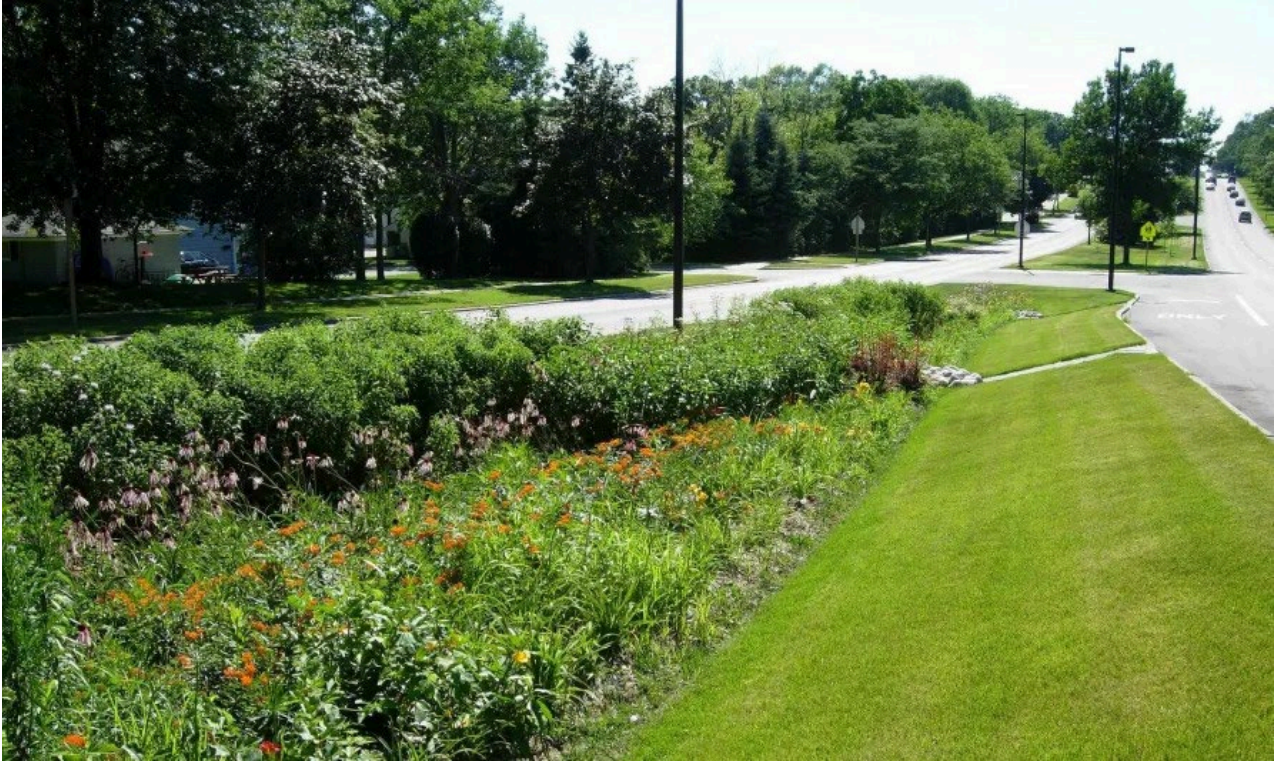
Figure 3.16: Bioretention cell with planting
