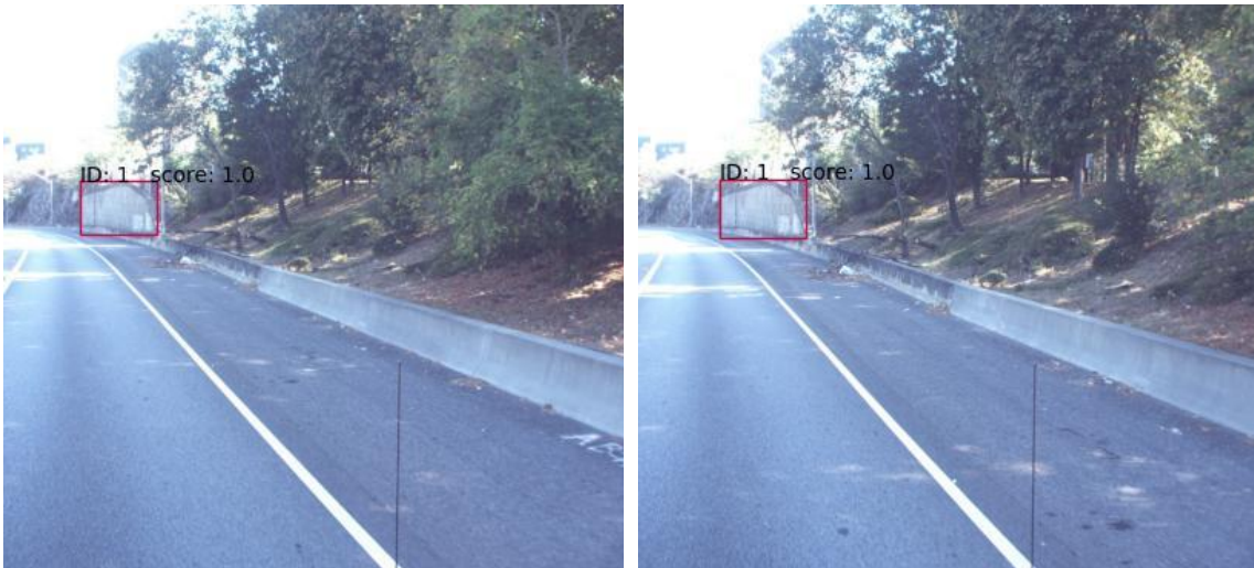
Figure 66. Photo. Tracking to cluster the same retaining walls at different roadway images.
