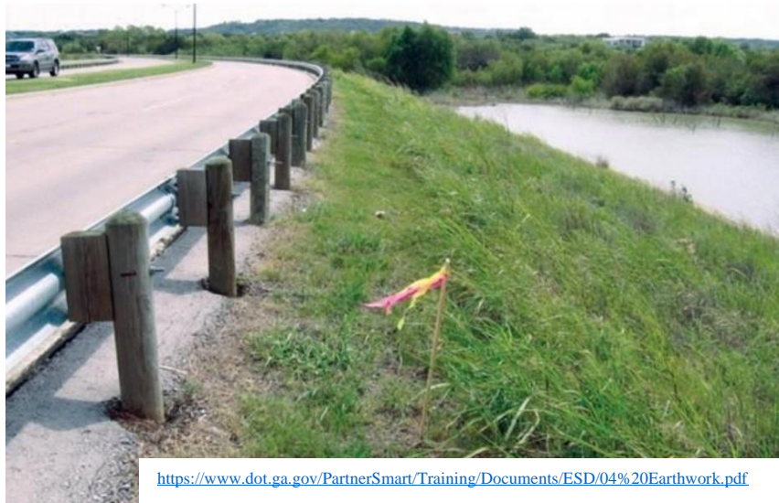
Figure 7. Photo. Embankments as part of the transportation network in Georgia.
