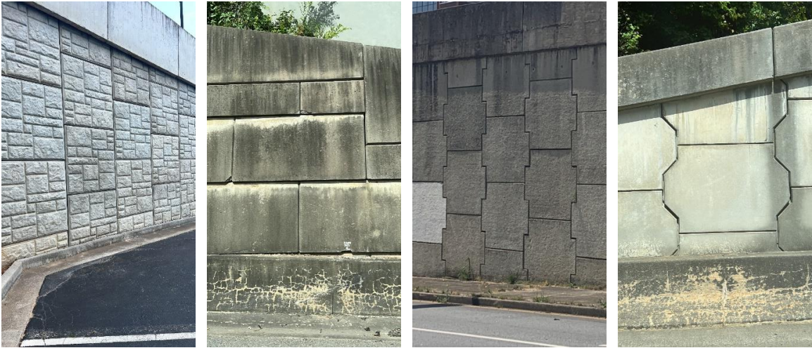
Figure 59. Photo. Examples of four types of retaining wall panels (from left: square, rectangle, cruciform, and Georgia-cruciform).
