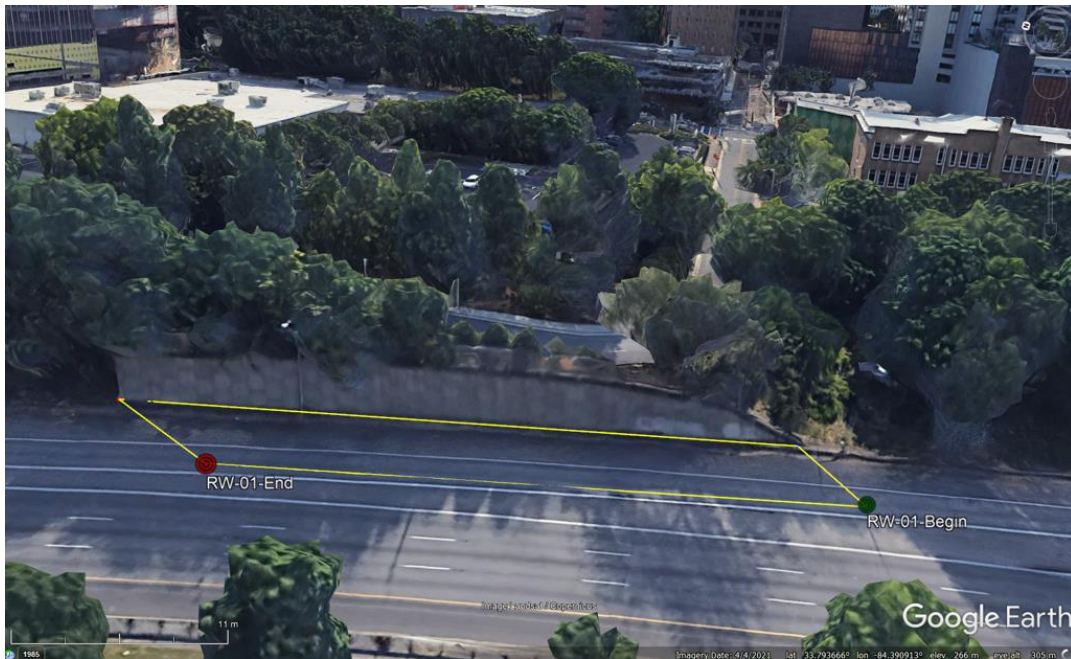
Figure 72. Photo. Discrepancy of retaining wall length measurements.
