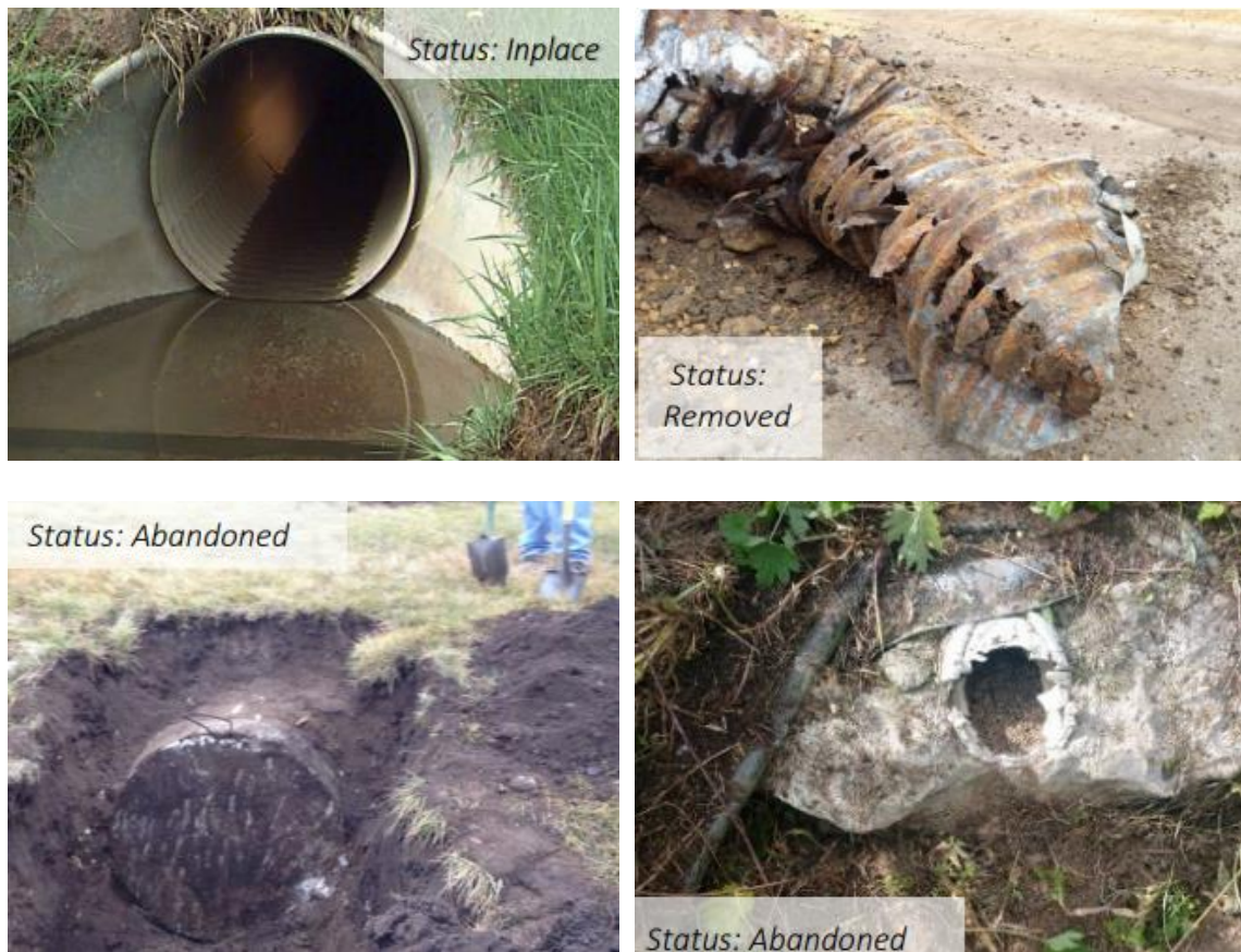
Figure 12. Photo. Status of culvert assets ( MnDOT, 2021b ).
