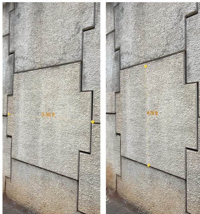
Figure 62. Photo. Displaying measurements using Filio.
