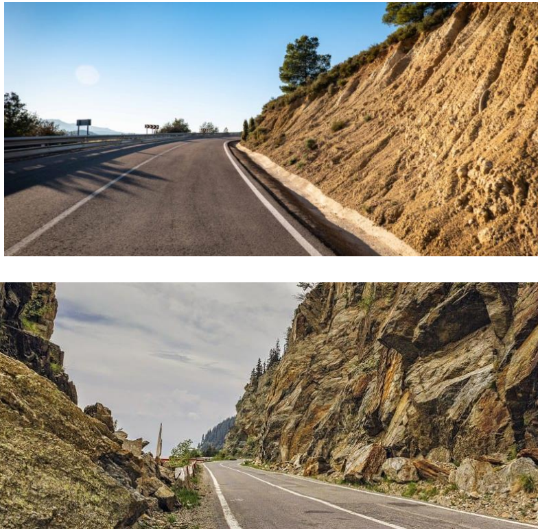
Figure 6. Photo. Soil and rock cut slopes as slope assets ( Beckstrand, 2017c ).
