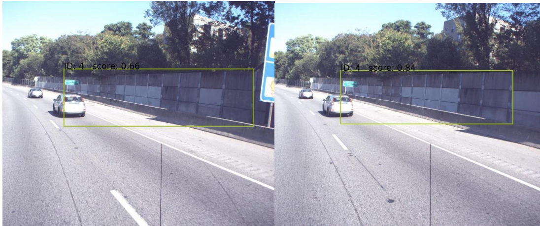
Figure 70. Photo. Examples of falsely recognized noise barriers as retaining walls (FP case).
