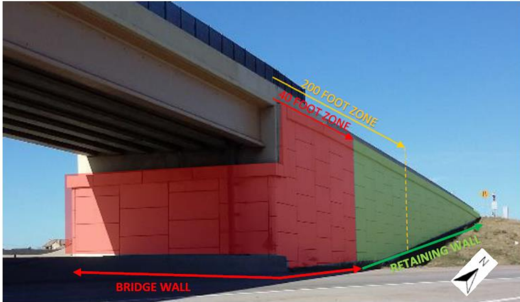
Figure 40. Photo. Bridge wall zone, scenario 03 (Walters et al., 2016).
