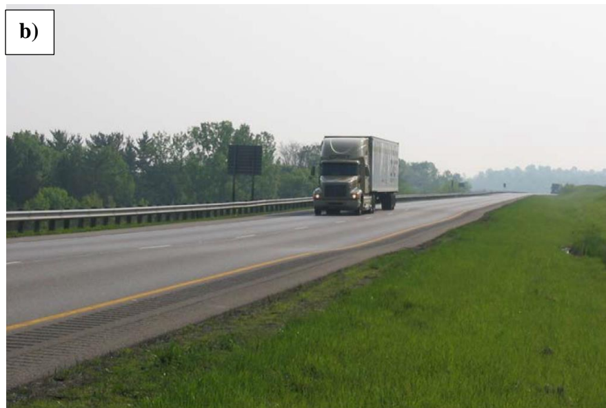
Figure 24. Photo. Example of a Class B embankment-slope: Downslope does not represent a safety risk, but the dip in the roadway is perceived, affecting serviceability and demanding the intervention from the Operation & Maintenance Office. Roadside ditches should always be clean and obstruction-free to achieve flawless drainage conditions. Moreover, a timely report accompanied by a proper condition assessment might prevent the downslope from going from a fair condition to a poor one (ODOT, 2013).
