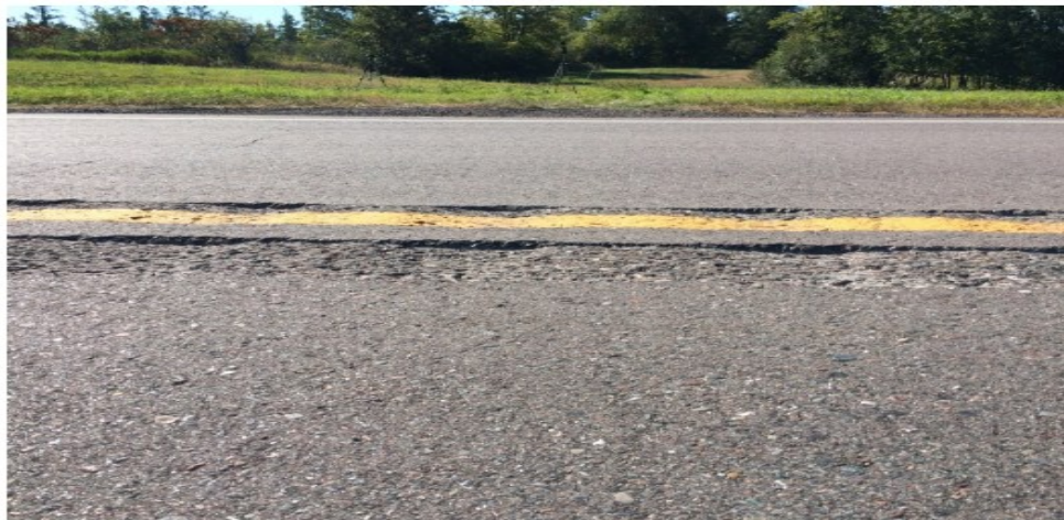
Figure 2.7: Sinusoidal rumble strip design from MNDOT optimization study (Terhaar et al. 2016)
