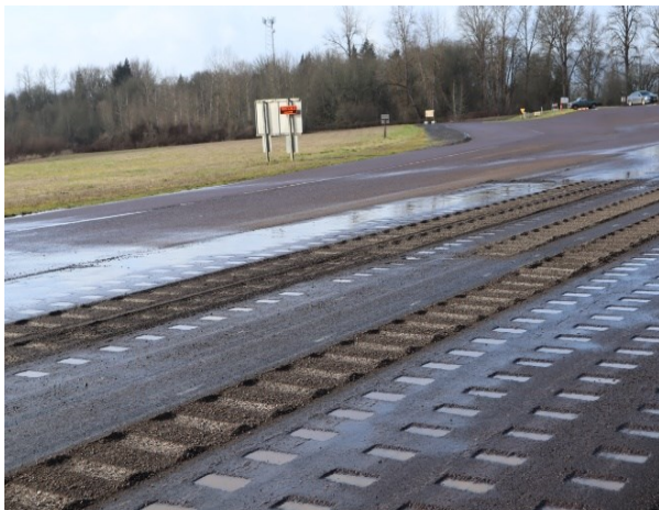
(e) Section during CLRS milling (2/26/2021)
