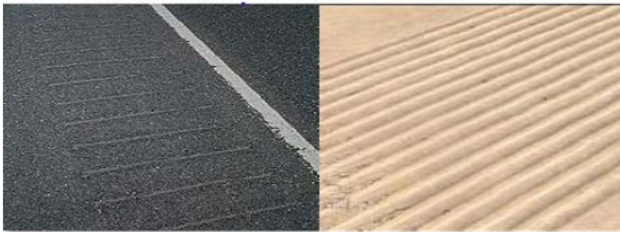
Figure 2.4: Rolled or formed rumble strips (Richards & Saito, 2007)(Guin et al. 2014)
