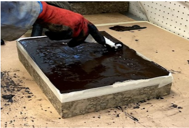
(c) Spreading emulsion
