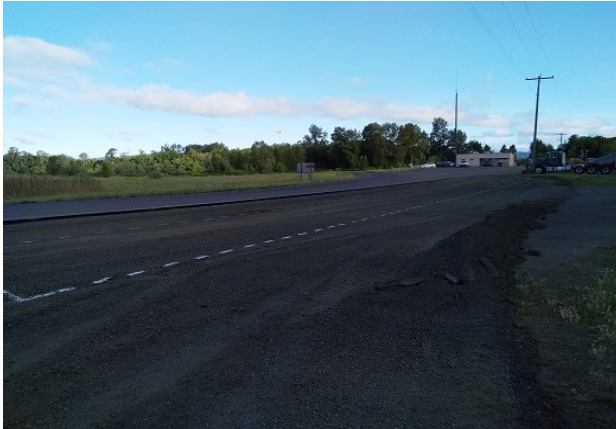
(a) Section before construction (6/25/2020 – 7am)
