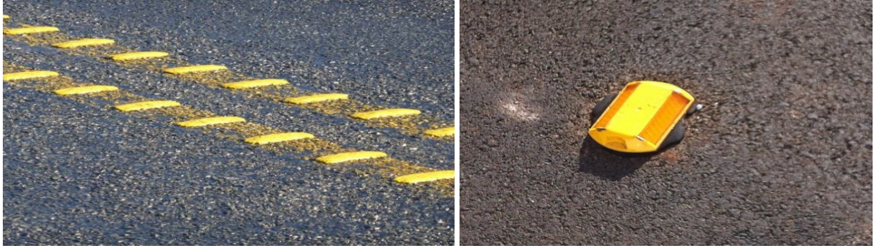
Figure 2.6: Raised rumble strips and pavement markers (Cottingham, 2020) (Raised Pavement Markers, 2020)
