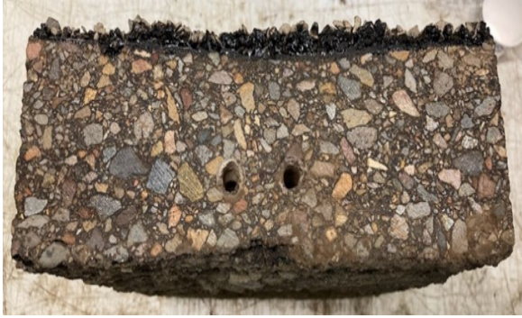
(a) Holes drilled
