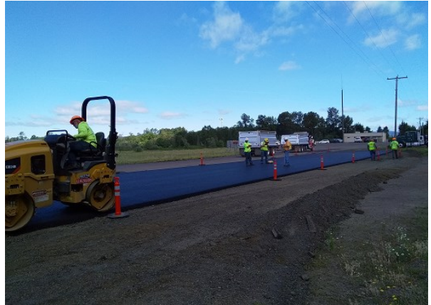
(b) Section construction (6/25/2020 – 12pm)
