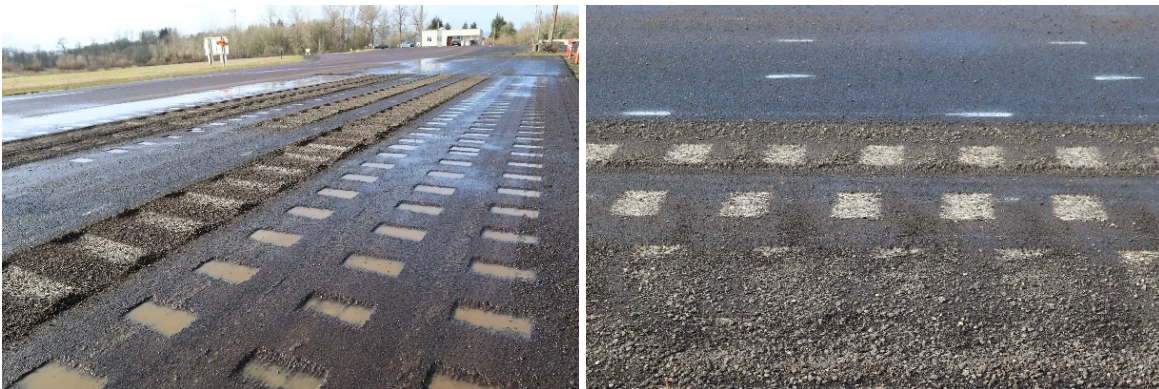
Figure 2.5: Examples of milled rumble strips from the Oregon State University test section
