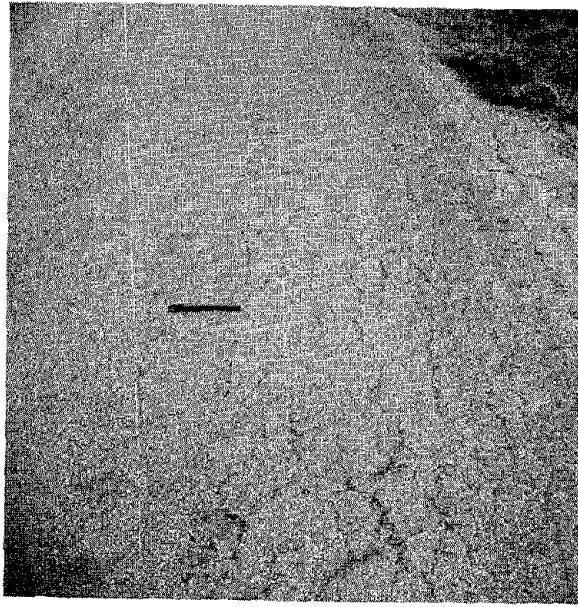
Class 2 Cracking
