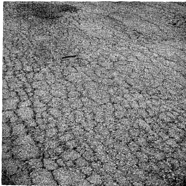
Class 3 Cracking
