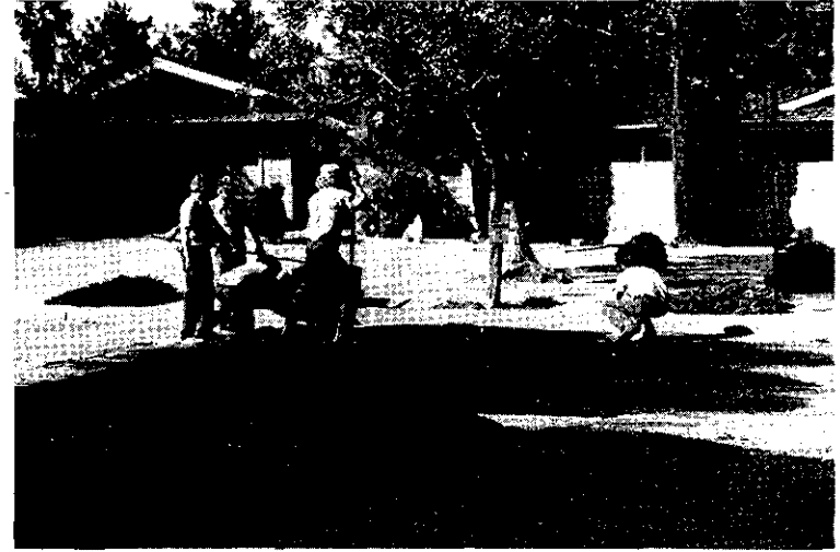
Using the template as a spreading device.
