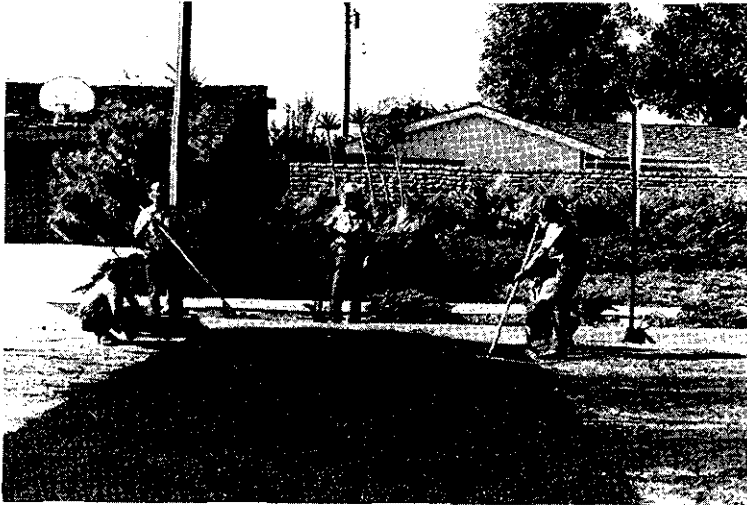
Laying the AC material. A 2x12 board inscribed with the hump shape service as a template.
