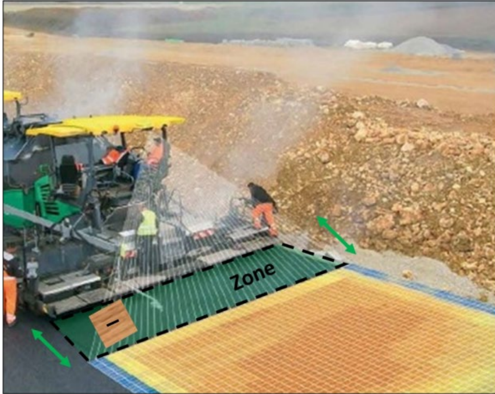
Figure 26. Illustration. Example of placing the event marker directly behind the screed.
