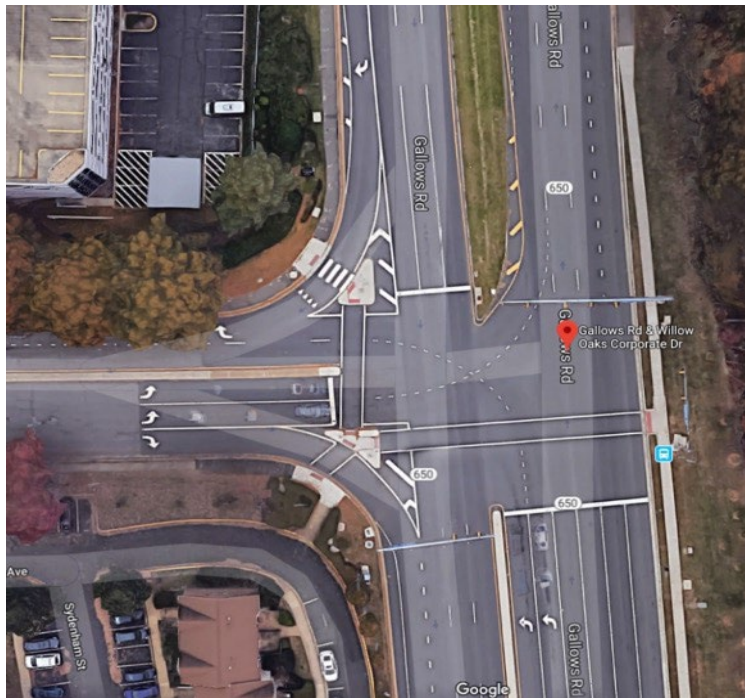
Figure 4. Photo. Intersection at Gallows Road and Willow Oaks Corporate Drive.
