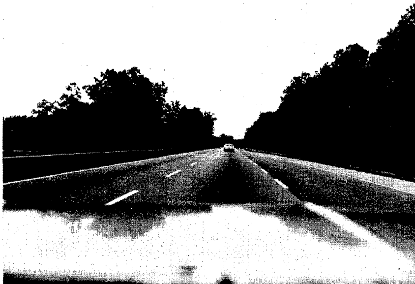
Figure 31. Pavement Markings Separating Acceleration Lane from Through Lanes.
