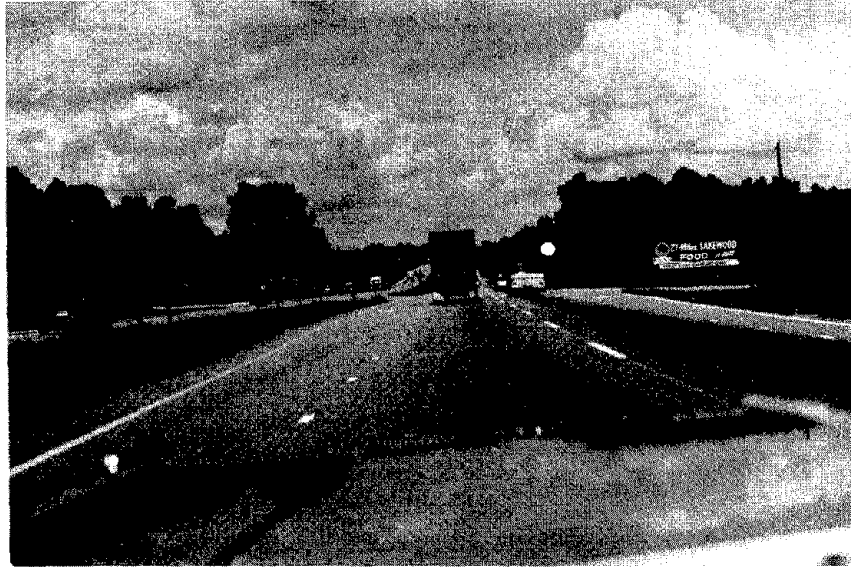
Figure 34. Pavement Markings Separating Turn Slots From the Through Lanes (Heavier Markings are Recommended).
