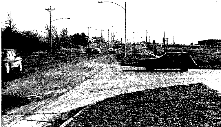
Figure C-12.1 - Right-Turn Acceleration Lane
