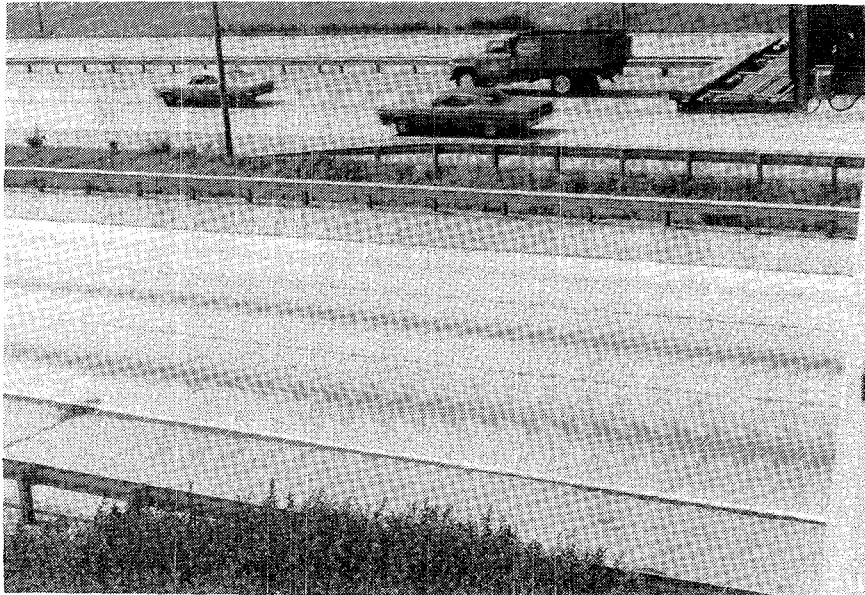
Figure 6.3. CRCP-2, Continuously Reinforced Concrete Pavement.
