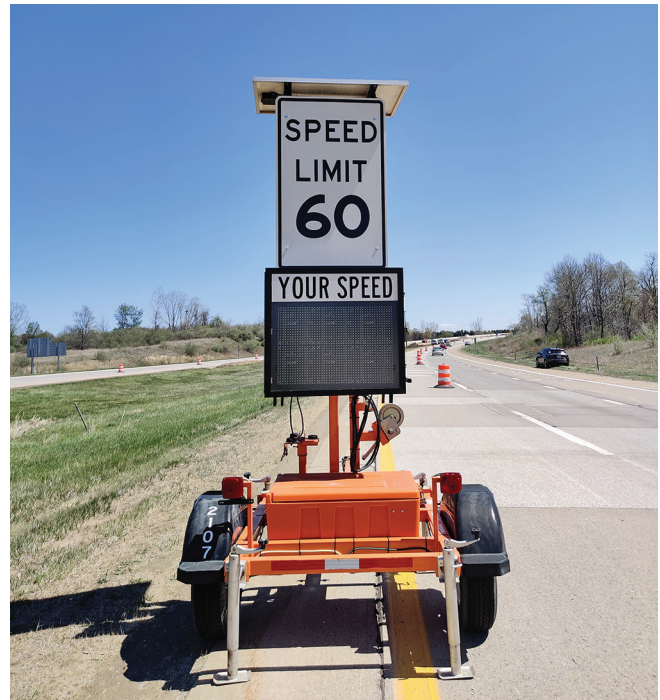
Speed feedback trailer at a work zone lane closure
