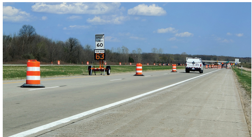
Speed feedback trailer positioned at the end of lane closure taper on westbound I-69 work zone in Michigan
