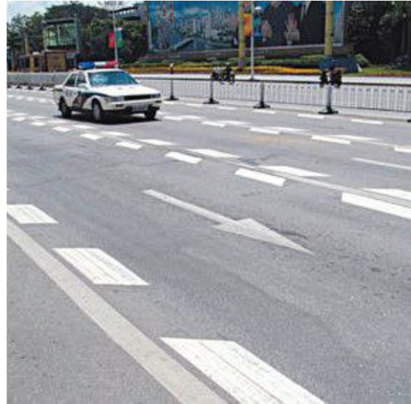
Figure 2.9 Longitudinal speed reduction markings.
