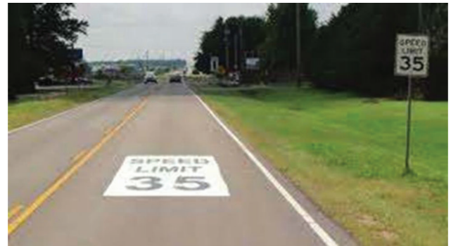
Figure 2.6 Speed limit pavement legend.
