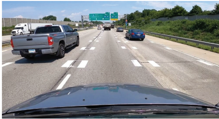
Figure 4.4 Longitudinal speed reduction markings on I-65 NB in Greenfield District.
