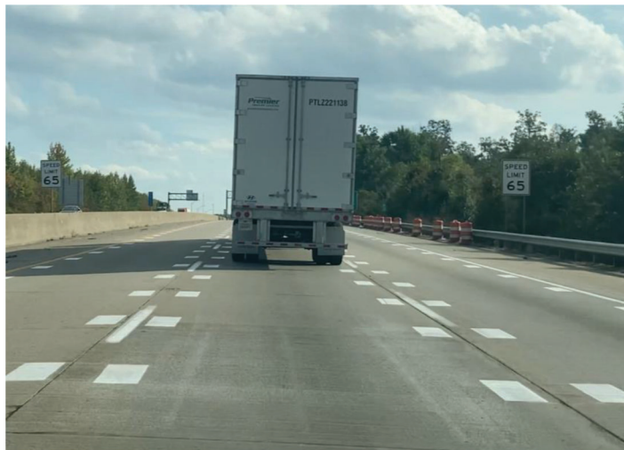
Figure 4.5 Longitudinal speed reduction markings on I-65 SB in Seymour District.
