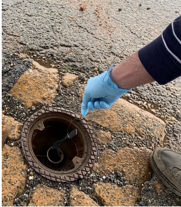
Figure C7. Deployment of gasket samples in the monitoring well.
