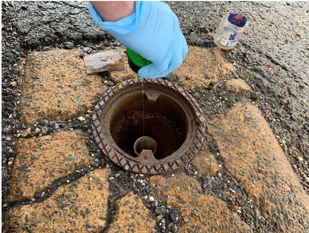
Figure C5. Installation of capsules in the well. Capsules are hung from the well's cap.
