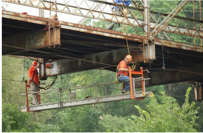
Figure A.1: Figure A-1. Scaffolds [78].
