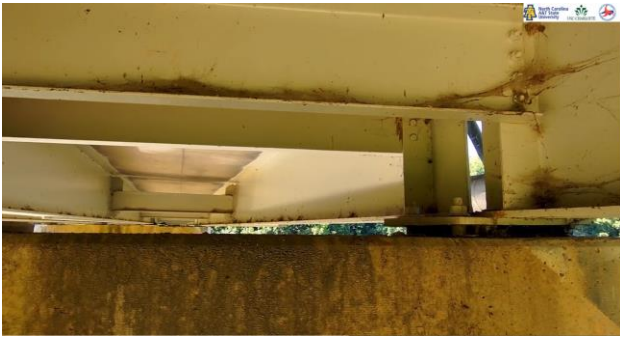
Figure 7.8: Diaphragm with bolted and welded connections shown, along with condition of concrete pier cap. Condition of bearing pad, plate, and bolts can also be observed.
