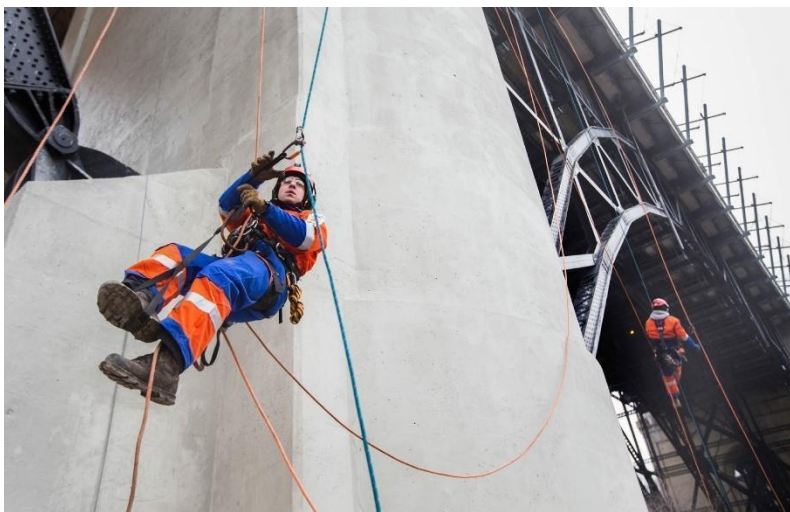
Figure A.3: Rope access [80].
