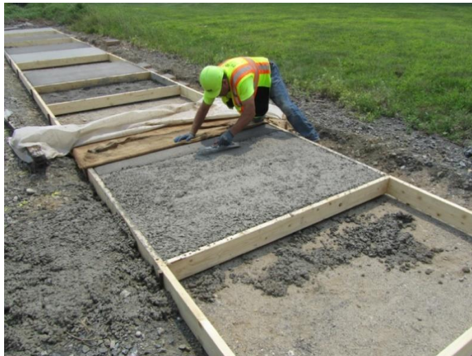
Figure 5.5 Worker uses trowel on concrete panel
