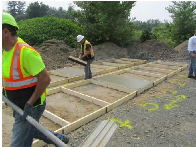
Figure 5.6 Worker using brush push broom to finish the surface of the panel
