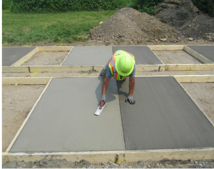
Figure 2.2 Worker trowels sidewalk panel following MassDOT specifications
