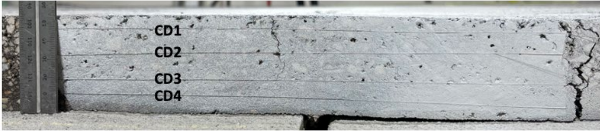
Figure 44. Photo. Non-interstate control scenario: cross-section after testing.
