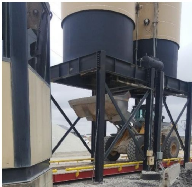
Figure 13. Photo. Filling a front wheel loader with an asphalt mixture at a plant.
