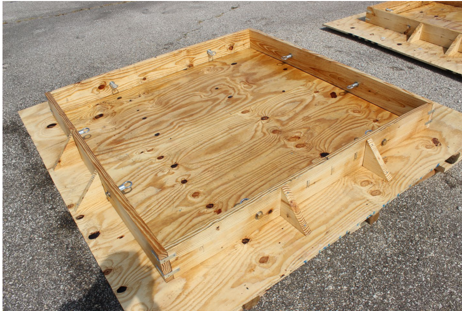
Figure 90. Photo. Wood forms with ferrule loops.
