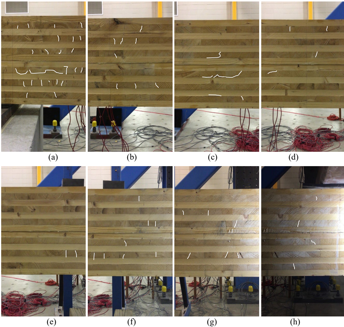
Figure 2.82 Southeast sections of CLT girder after the testing captured by manipulator: (a) section 1; (b) section 2; (c) section 3; (d) section 4; (e) section 5; (f) section 6; (g) section 7; and (h) section 8.
