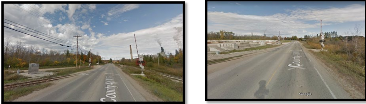
Figure 33. HRI 1 (Left) and HRI 2 (Right) Instrumented with RCVW and Active Warning Devices (Lights and Gates) (Photo Courtesy: Google Maps)
