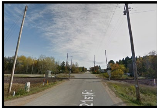
Figure 34. Baseline HRI 4, Active Warning Devices (Lights and Gates) (Photo Courtesy: Google Maps)
