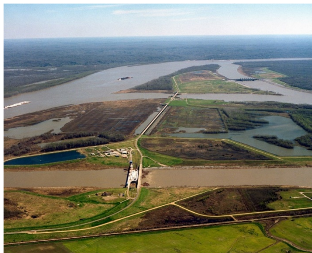
Figure 22. The Old River Control Structure complex—view is to the east-southeast, looking downriver on the Mississippi, with the three dams across channels leading to the Atchafalaya River to the right of the Mississippi
