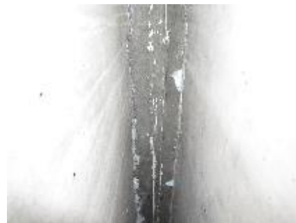
b. After Testing – Beneath Bridge
