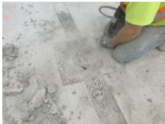
e. Pocket Demolishing
