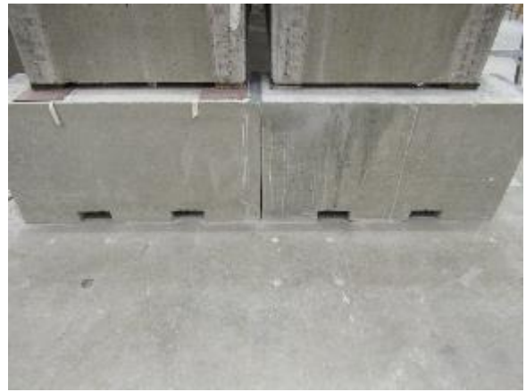
b. Placement on Abutment
