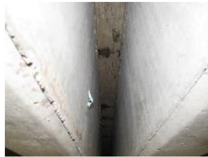
b. Leak in LMC after Fatigue Testing
