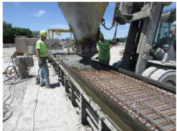
b. Concrete Casting
