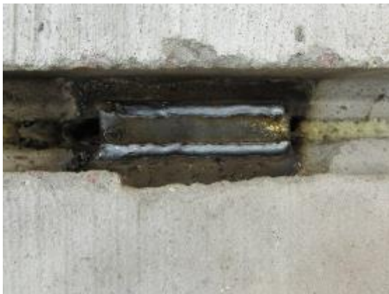
a. Welding Steel Plate to Angles Embedded in Girders
