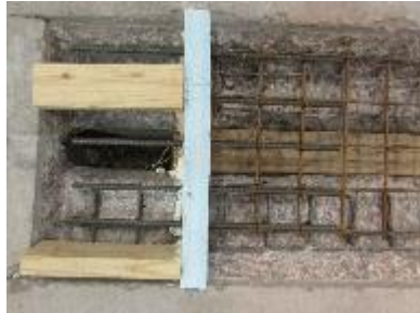
c. Block-out Formwork
