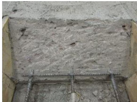
d. Roughened Joint Surface
