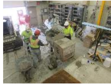
d. Mixing UHPC
