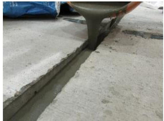
b. Grouting Girder-to-Girder Keyway
