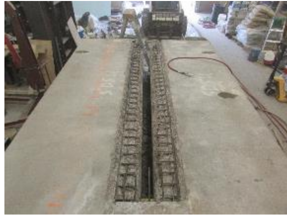
b. Continuous Joint Preparation – Segment II
