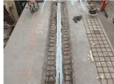
d. Continuous Joint Segment II Formwork
