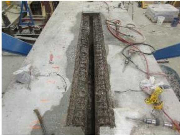
a. Continuous Joint Surface Preparation – Segment I
