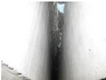
a. Before Testing – Beneath Bridge
