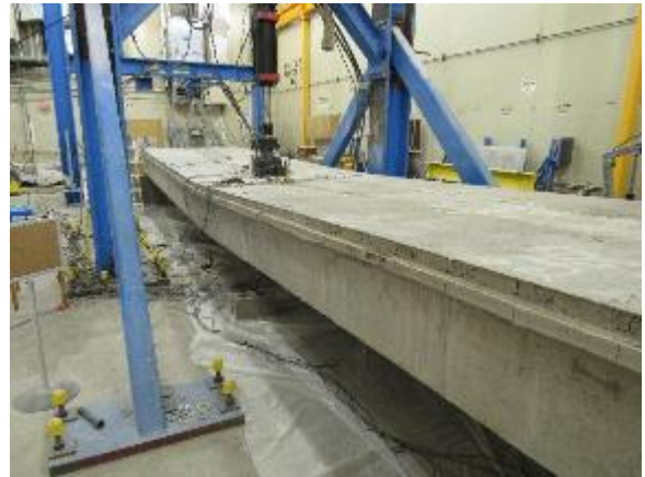
d. Bridge Condition at Failure
