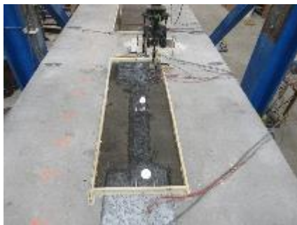
c. Before Testing – Top of Bridge
