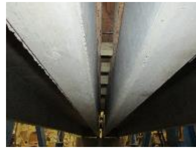
b. Underneath View, Continuous Joint Segment I Formwork
