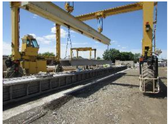
d. Removal from Formwork
