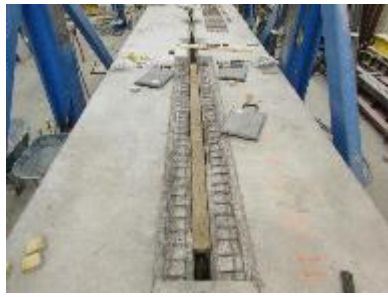
a. Top View, Continuous Joint Segment I Formwork
