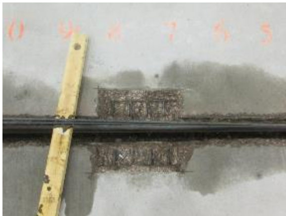
c. Pocket Joint and Intermediate Keyway
