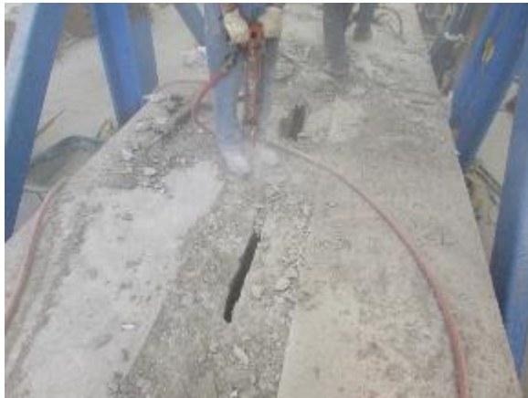
c. Continuous Joint Demolishing – Segment I
