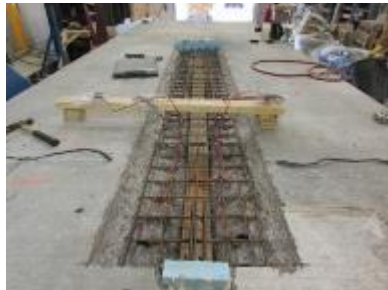
e. Continuous Joint Reinforcement
