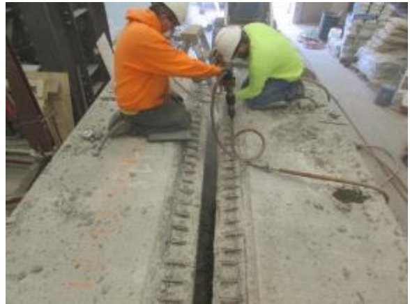
d. Continuous Joint Demolishing – Segment II
