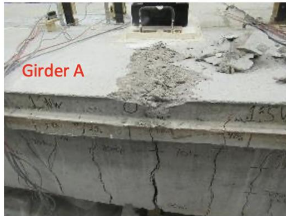
c. Compressive Failure of Concrete at 9.5-in. Deflection
