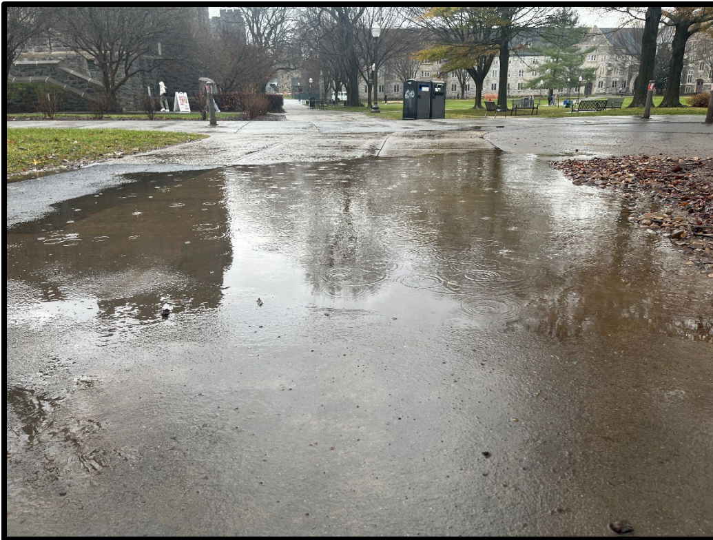
Figure 3. Path blocked by pooled rainwater.
