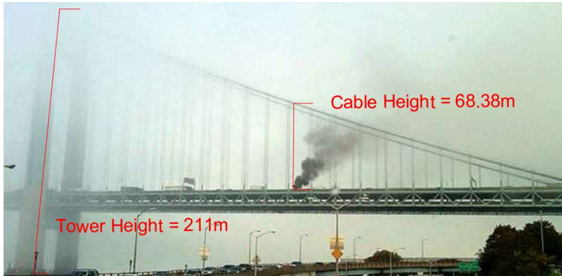
Figure 64 - Truck fire on the Verrazano-Narrows Bridge, New York (Berke).
