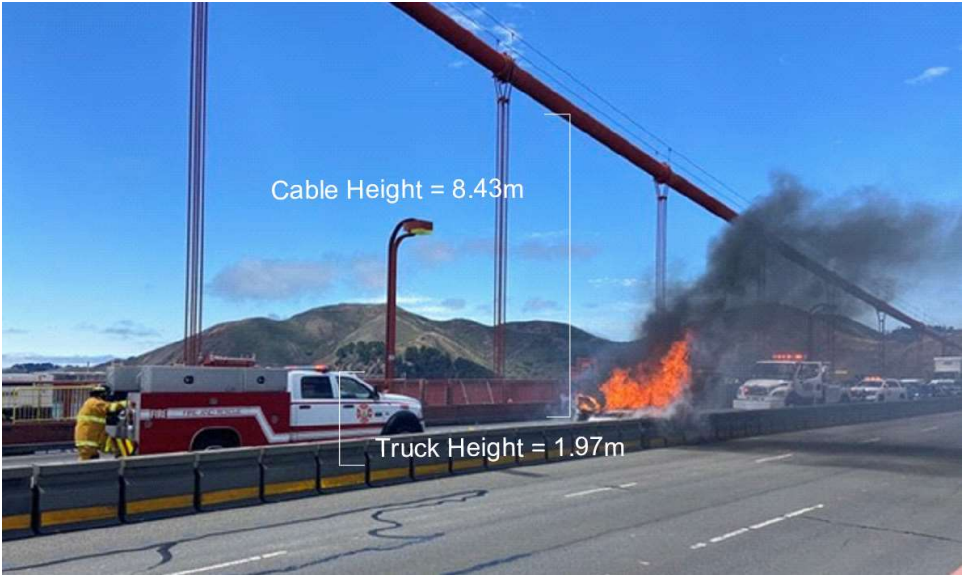
Figure 62 - Car fire on southbound Golden Gate Bridge, California (CBS San Francisco).
