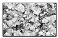
Figure 4 Typical Consequences of Pavement Markings Impacted by Roadway Surface Characteristics (Poor Material Coverage on Backside of Aggregate)
