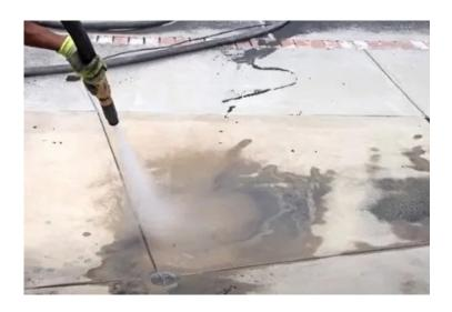
Figure 62 Sandblasting Equipment for Surface Preparation
