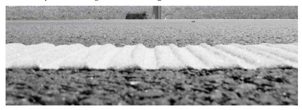
Figure 25 Typical Inverted Profile Thermoplastic Marking (Profile View)
