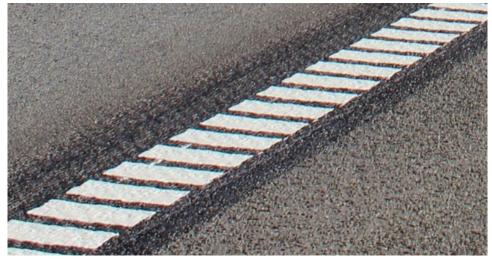
Figure 31 Extraction Profiled Marking Application Method-Long Flex Line
