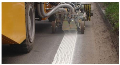
Figure 30 Dot Profile Marking Application Method
