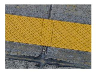
Figure 21 Preformed Tape (MnDOT, 2015)
