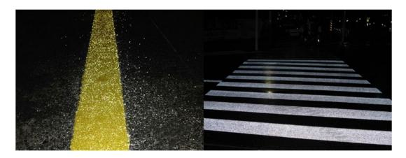
Figure 32 All-Weather Thermoplastic Retro-reflectivity During the Night (Source: Yeng Hsingh Co., Ltd, 2020)
