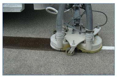
Figure 74 Water Blasting Paint Removal Equipment
