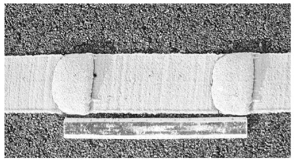
Figure 26 Typical Raised Profile Thermoplastic Marking (Overhead View)
