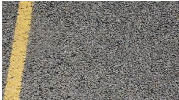
Figure A-505. SH0029-1, Inside WP.
