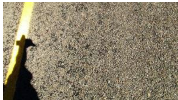
Figure A-481. SH0029-3, Inside WP.
