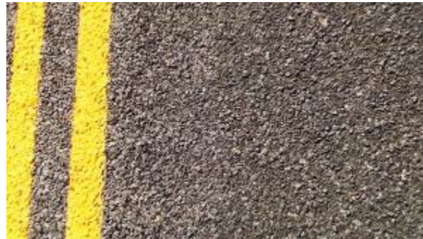
Figure A-64. SH0092-4, Inside WP.
