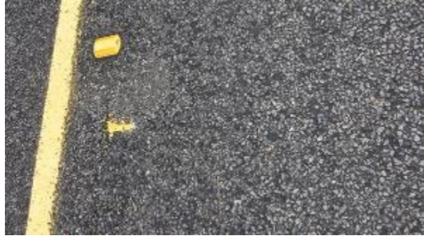
Figure A-926. SH0289-4, Inside WP.
