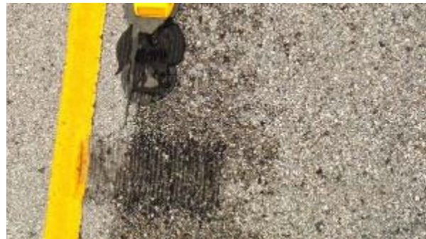
Figure A-868. SH0289-1, Inside WP.
