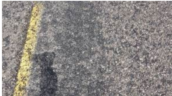
Figure A-365. SH0070-6, Inside WP.
