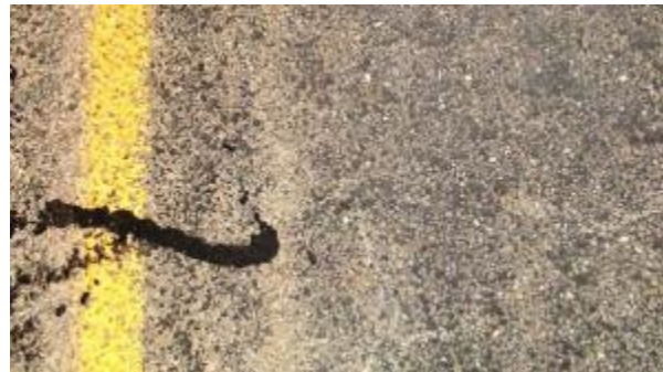
Figure A-36. SH0092-1, Inside WP.
