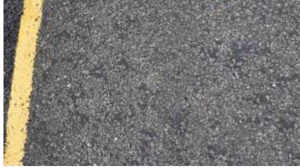
Figure A-918. SH0289-2, Inside WP.
