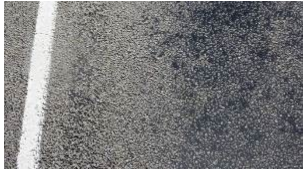
Figure A-549. SH0029-6, Inside WP.
