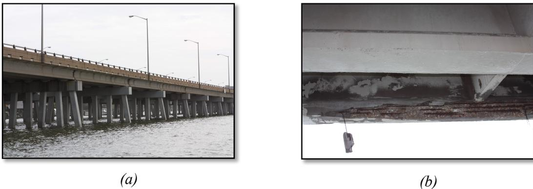
*Figure 1 – Hampton Roads Bridge Tunnel (a) approach span and (b) deterioration*
