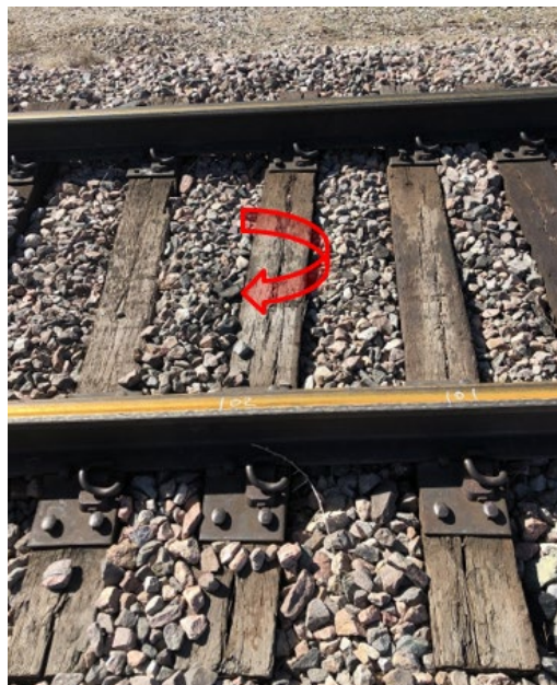
Figure 31. Timber Crosstie Skew Example
