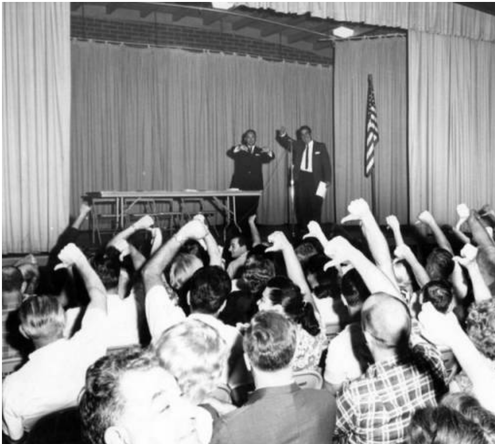
Figure ES-4. Anti-freeway Protest Meeting of Valley Homeowners, to the West of Pacoima
