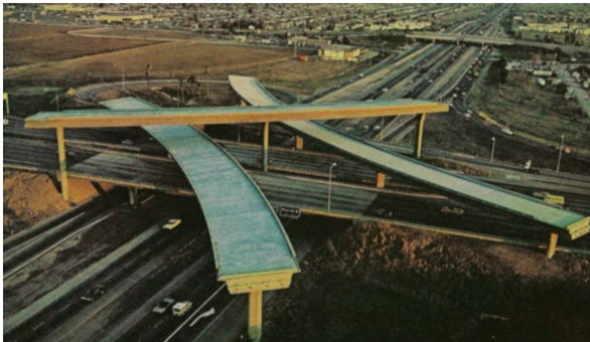
Figure 8-12. Unfinished US-101/I-280/I-680 Interchange, 1976
