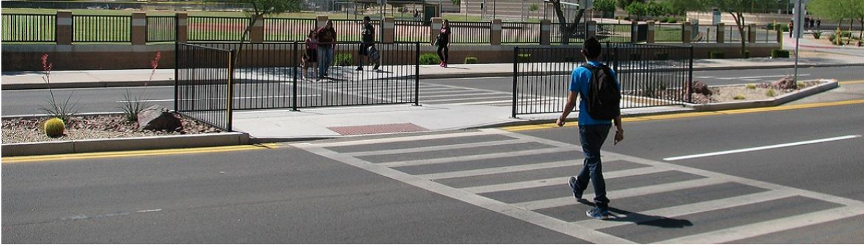
Figure A-14 Crossing Island with Fencing (AASHTO)
