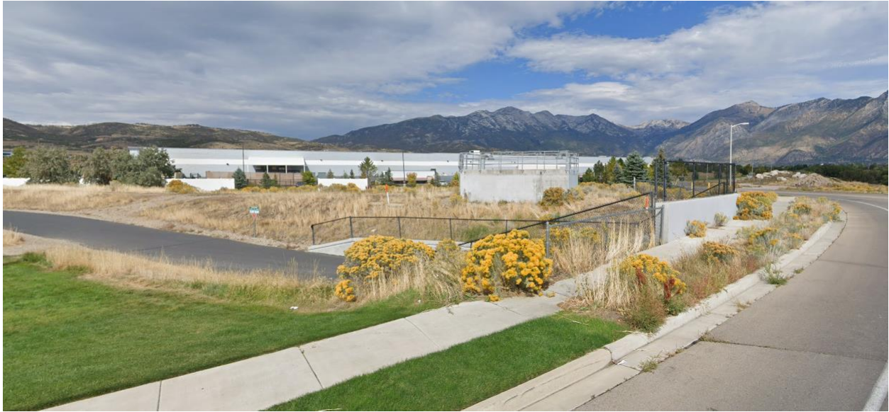
Figure A-10 Bike Path Crossing Beneath Grade: Lehi, UT
