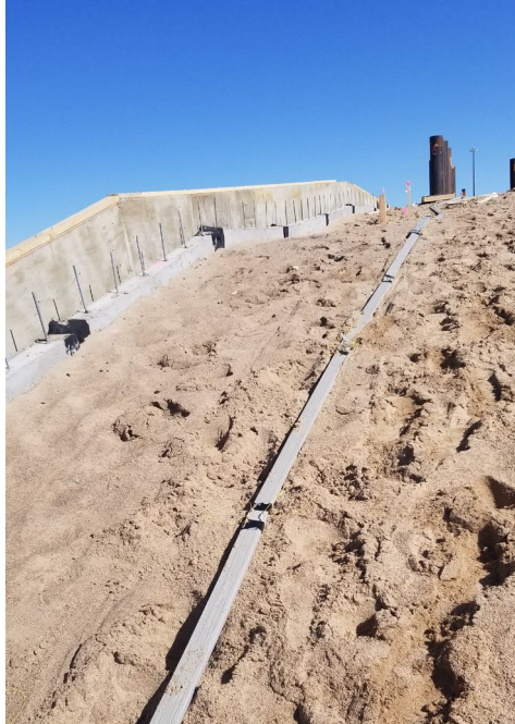
(a) extended composite beams for one pile (b) anchors on the center of each beam
