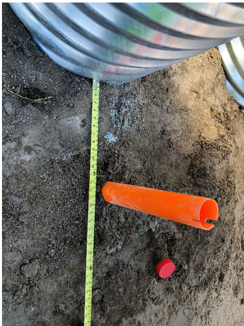
(c) distance between CMP sleeves and casing
