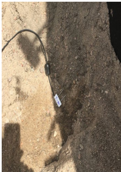
(a) moisture sensor embedded in the backfill
