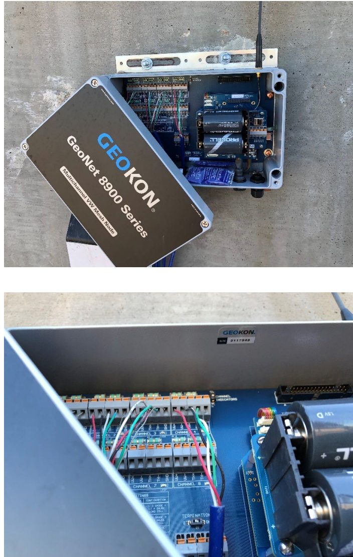
Figure 3.46: Interior view of the south abutment and its wiring scheme
