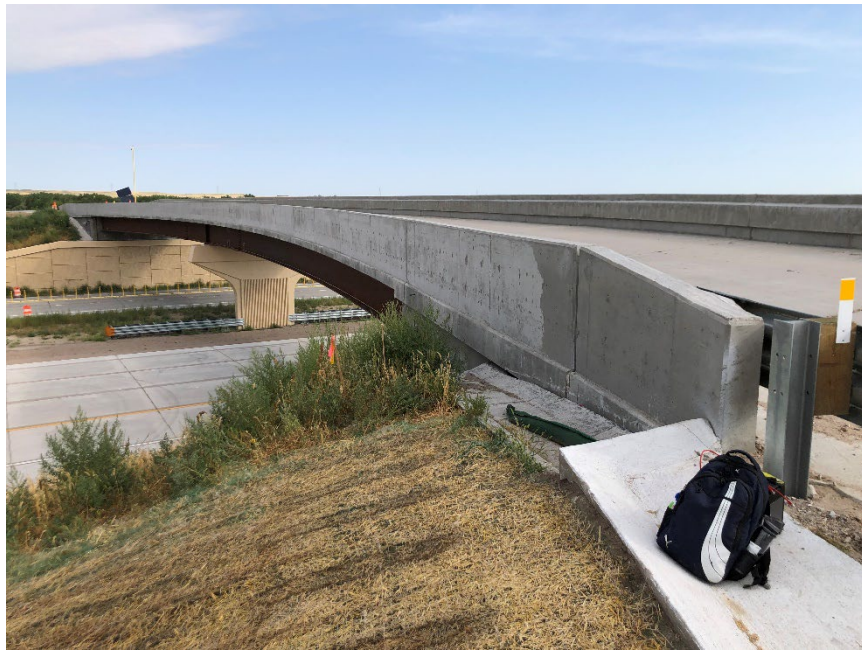
Figure 3.1: Big Springs Bridge (S080-10302) over I-80
