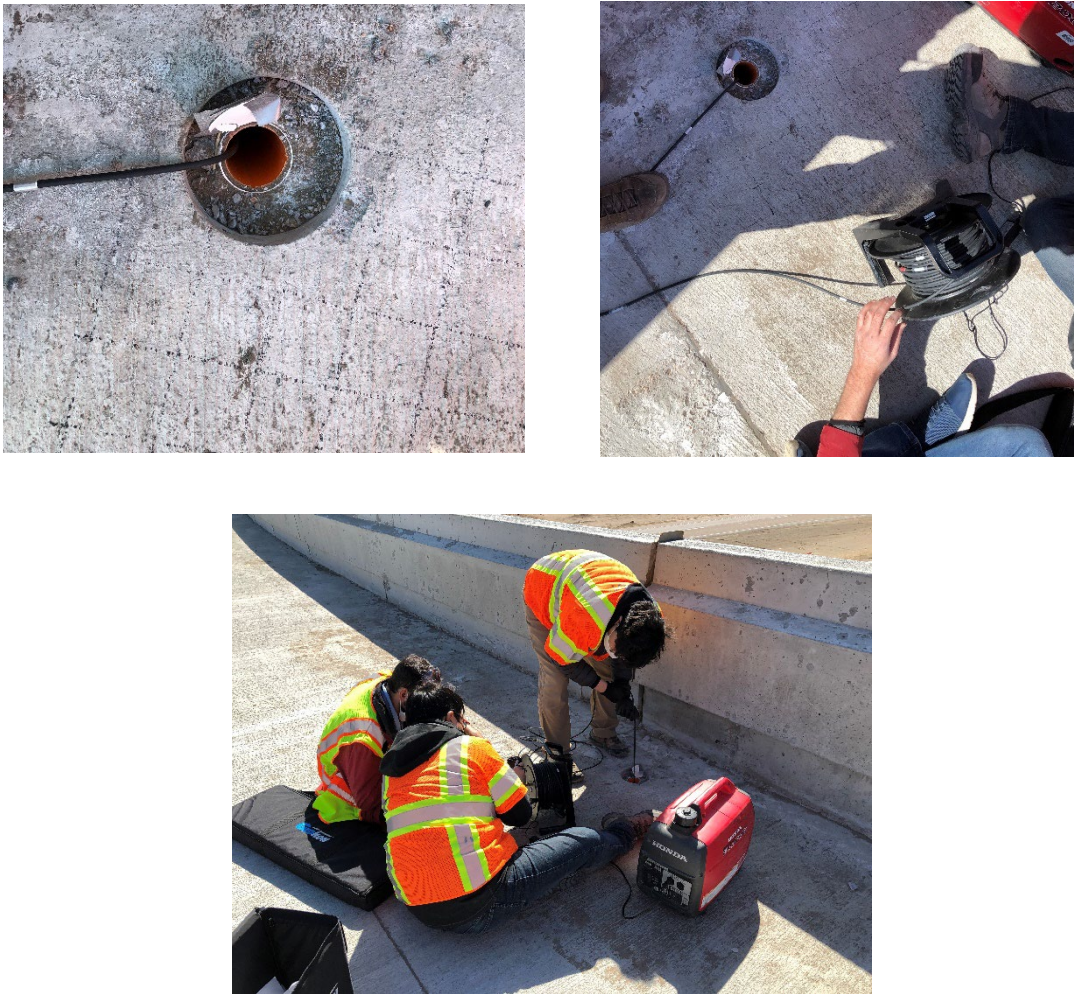
Figure 3.24: Taking Inclinometer Readings
