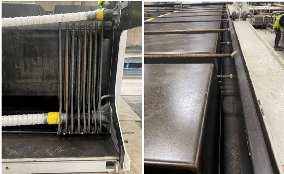
Figure 4.14: End zone reinforcement for PT specimen (left) and edge form with lip (right)
