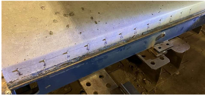
Figure 5.19: DEMEC gauges installed for strain measurements at girder end
