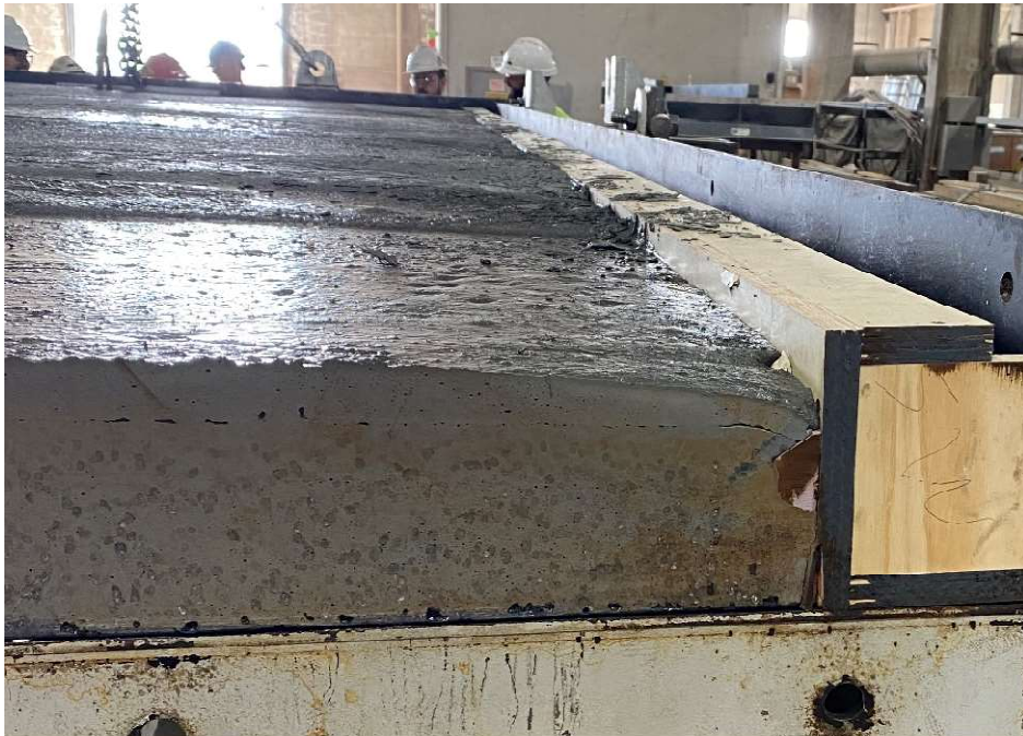
Figure 4.25: Unfilled corner of the form
