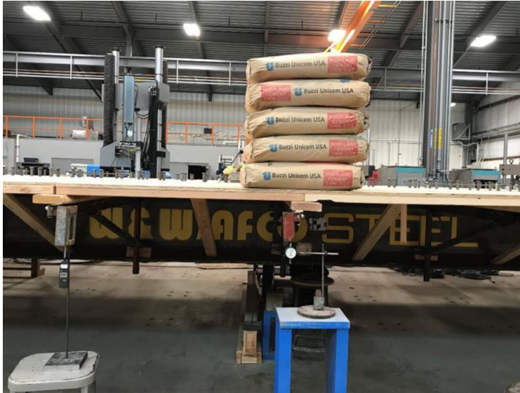
Figure 4.4: Cement sacks are being used to provide eccentric loading to the formwork and bracing systems in order to measure the load effects on temporary structures.
