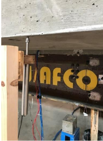
Figure 4.10: Installation of LVDT sensors at the midspan location of South Girder (LVDT 3) and South edge of slab overhang (LVDT 4)
