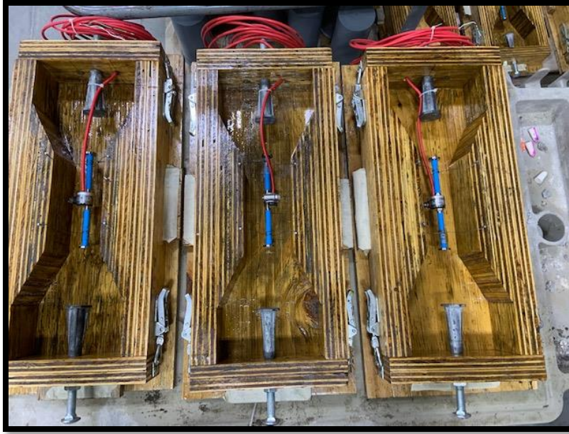
Figure 5.2 Dogbone Forms Prior to Casting with Vibrating Wire Gages Installed
