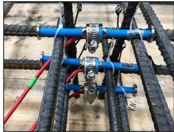
b) VWSG Location 2 at CL of Deck Slab
