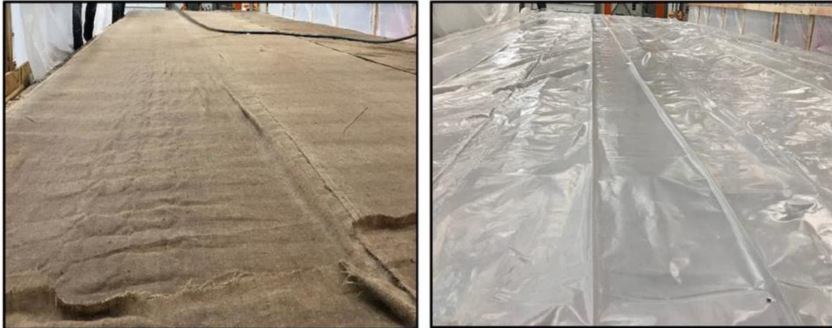
Figure 4.14: Wet burlap and 2 mil plastic was applied for 14 days
