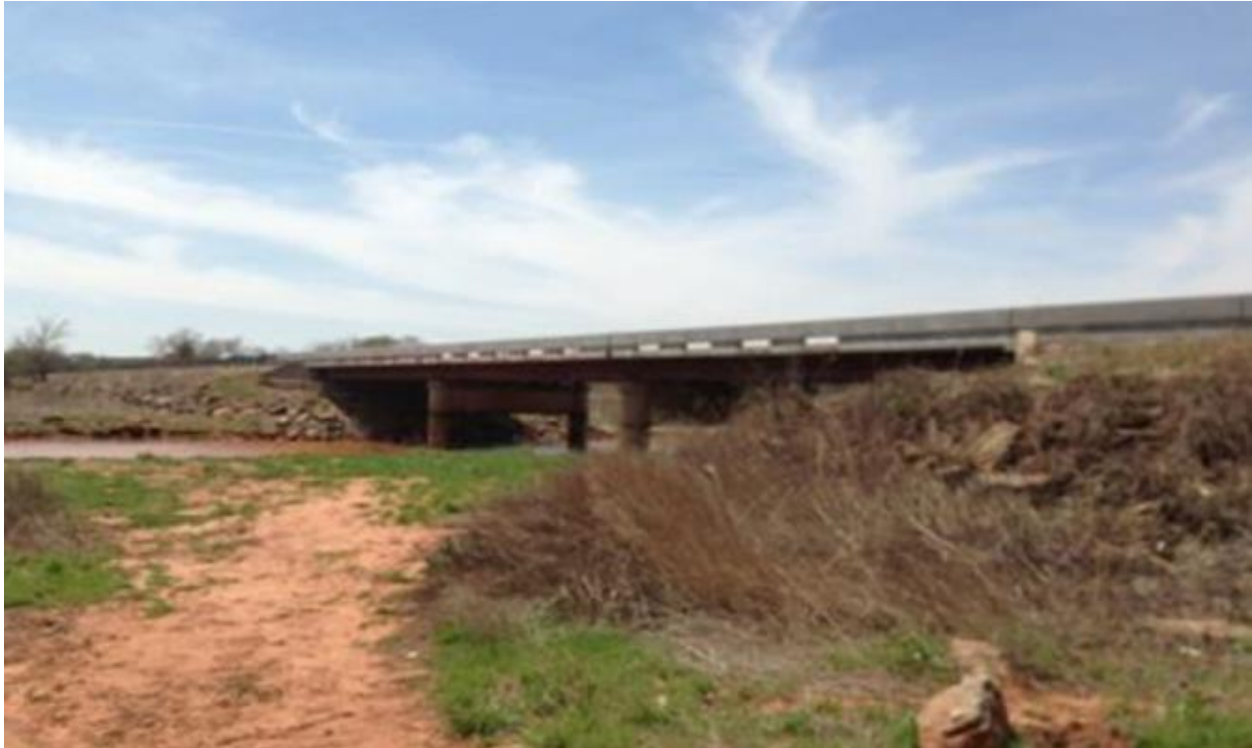
Figure 3.4 SH 86 over Stillwater Creek, Payne Co., Oklahoma, View Lkg SW
