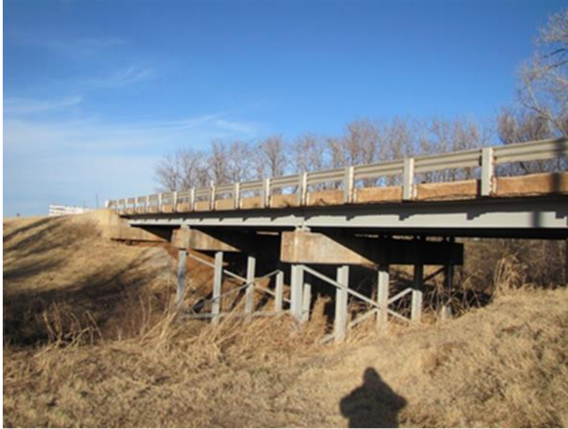
Figure 3.7 US 281 Bridge over Spring Creek, Woods Co., Oklahoma, View Lkg SW
